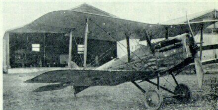
A8917, second of the two S.E.5's completed without armament. The drain bowls for the tanks in the centre-section leading edge can be seen in the \frac{3}{4} -front view; the overflow pipes are visible in the other.
