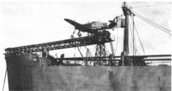
As the Battle of Britain drew to a close the delivery to the R.A.F. of Hurricane II's commenced and the surplus of Mark I's was allocated to numerous first line duties apart from metropolitan day defence. Perhaps most widely used were the Sea Hurricanes. Broadly speaking the main versions which had originated from the Mark I were the Sea Hurricane IA, with eight machine guns, catapult spools and no arrester hook, and the Sea Hurricane IC, with four 20-mm. Hispano guns, catapult spools and arrester hook (top two pictures, British Official Photos, Neg. Nos. 12194C and 12193C). The Sea Hurricane IB (third picture, Admiralty Neg. No. A18870) was an arrester-hooked version of the IA, this No. 801 Squadron aircraft being refueled aboard H.M.S. Argus. Sea Hurricanes IA were developed early in 1941 for convoy defence, being mounted on Catapult Aircraft Merchantmen (CAM-Ships) V6756 is shown here aboard S.S. Empire Tide in August 1941.
