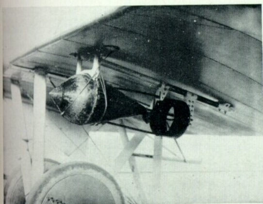
Left: The bomb rack for a single Carbonit bomb under the wing of a Gotha G.I. (Photo: W. Puglisi) Right: Gotha taken over by the Netherlands air service, seen here in Dutch markings in the L.V.A. workshops. The fin serial is 'LA 50'. (Photo: G. H. Kamphuis)
