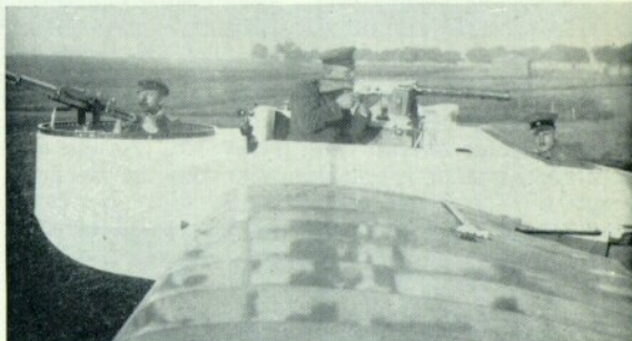
Oskar Ursinus demonstrating an early version of the 20 mm Becker cannon in the forward position of a G.I.
