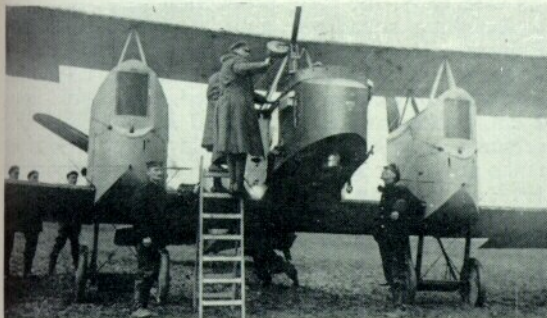
Left: Interested pilots of Jasta 4 examine Gotha G.III 397/16 at Marchais in May 1917. The slim fuselage and Cellon windows on the side of the front cockpit are here evident. Right: G.III 397/16; the passageway on the right side of the fuselage connects the front and rear cockpit; the rear gun is mounted on a lateral slide rail; and mudguards on the wheels prevent stones being thrown into the propeller arc. (Photos: W. Puglisi)
