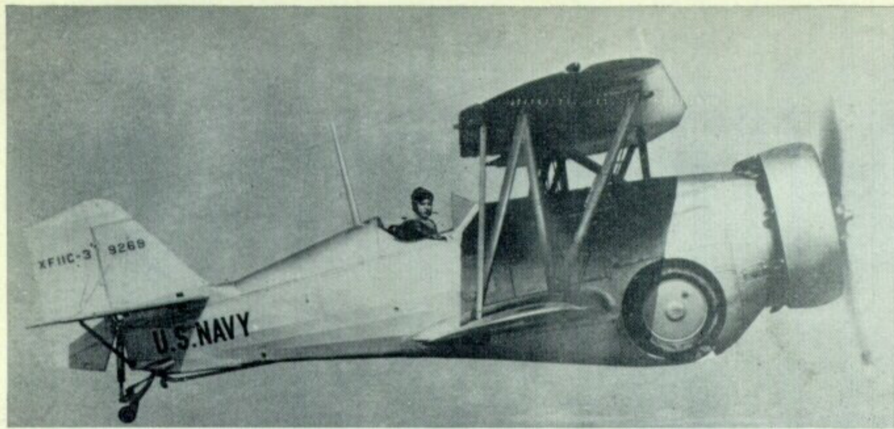
The XF11C-3 was converted from production F11C-2 serial 9269. (Photo: U.S. Navy)
