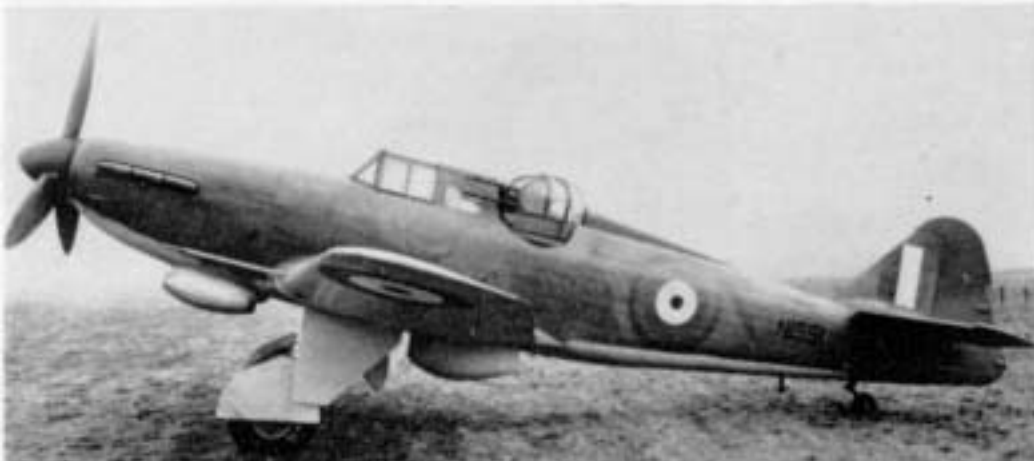
The Defiant Mk. II prototype N1550 at Boscombe Down in July 1942. Note deep radiator and retracted rear fuselage combing. (Photo: Peter Moss collection)
