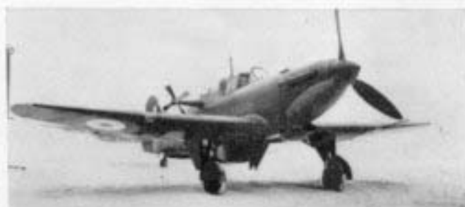
A Defiant Mk. II after conversion to the target-tow configuration; January 1942.
