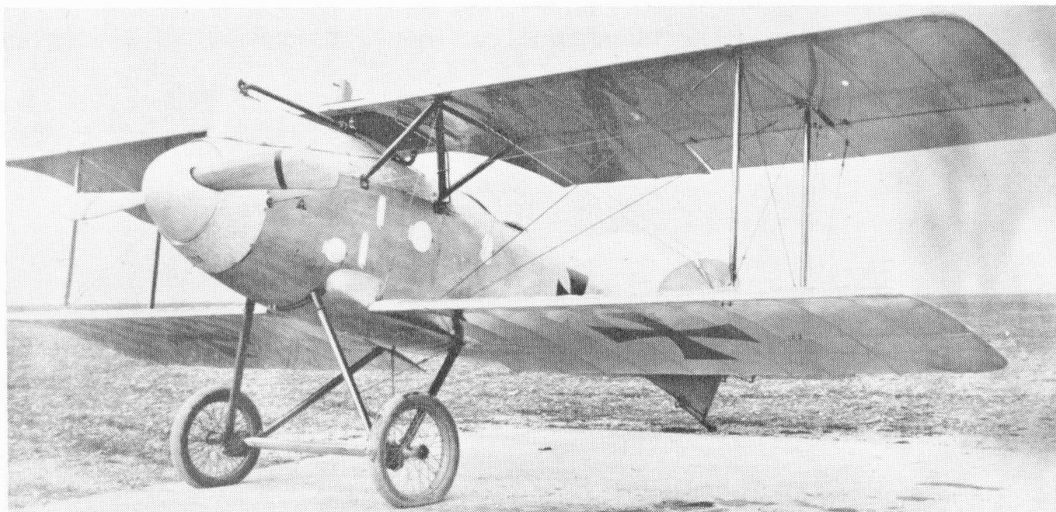
Later type of Albatros D II with flush radiator in centre of upper wing. The racier appearance resulting from the reduced gap is noticeable when compared with the D I. (Photo: Egon Krueger)
