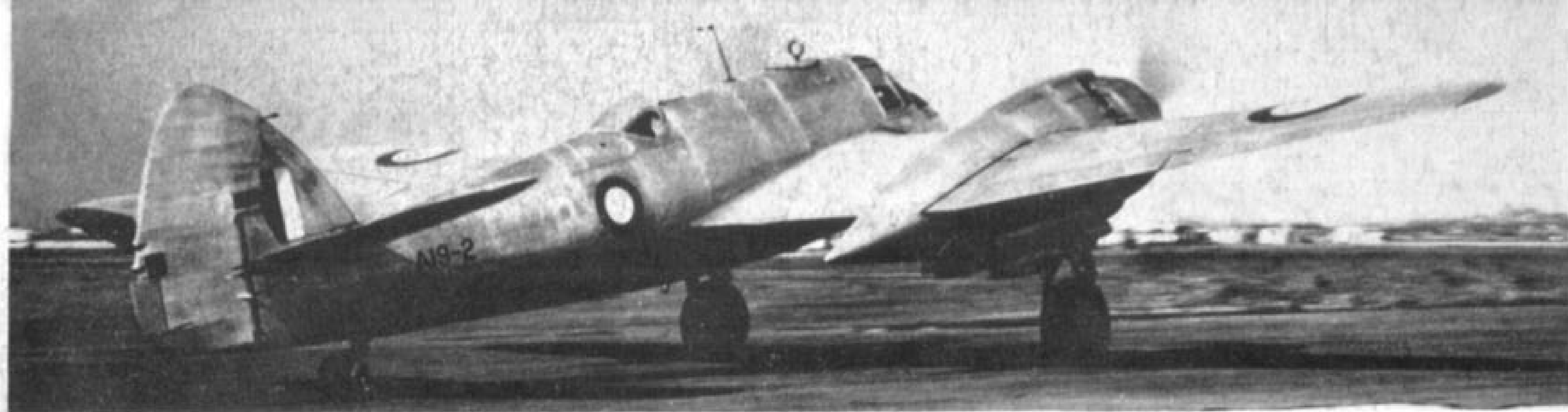
Two views of Fairey-built Beaufighter IC A19-2 in 1943 with Australian installation of Wright Cyclone GR2600-A5Bs in long nacelles for proposed production variants, Beaufighter VIII and IX.
