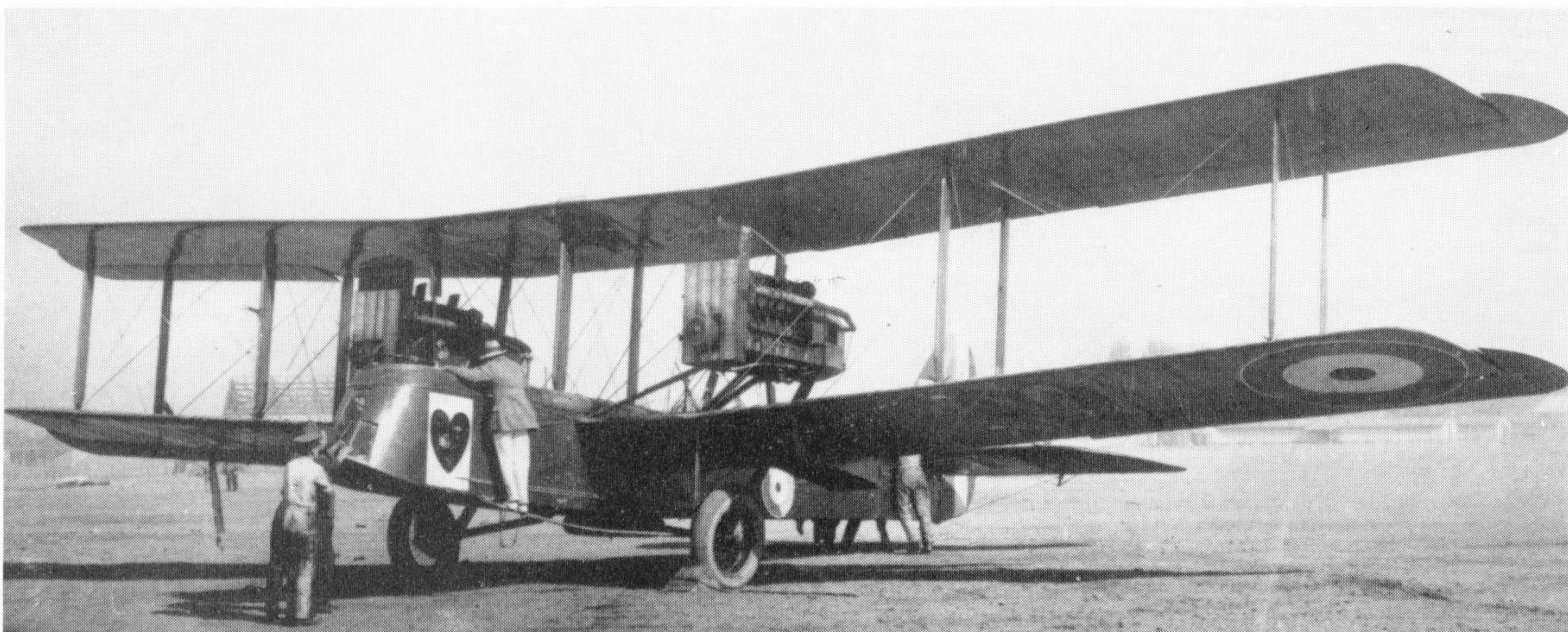
D.H.10 of No. 216 Squadron in Egypt in 1922. The aircraft has enlarged tropical radiators with shutters of the original length, and the engine cowling panels have been removed. At this time some of No. 216's D.H.10s bore markings of hearts, spades, clubs, diamonds and swastikas. (Photo: Ministry of Defence)
