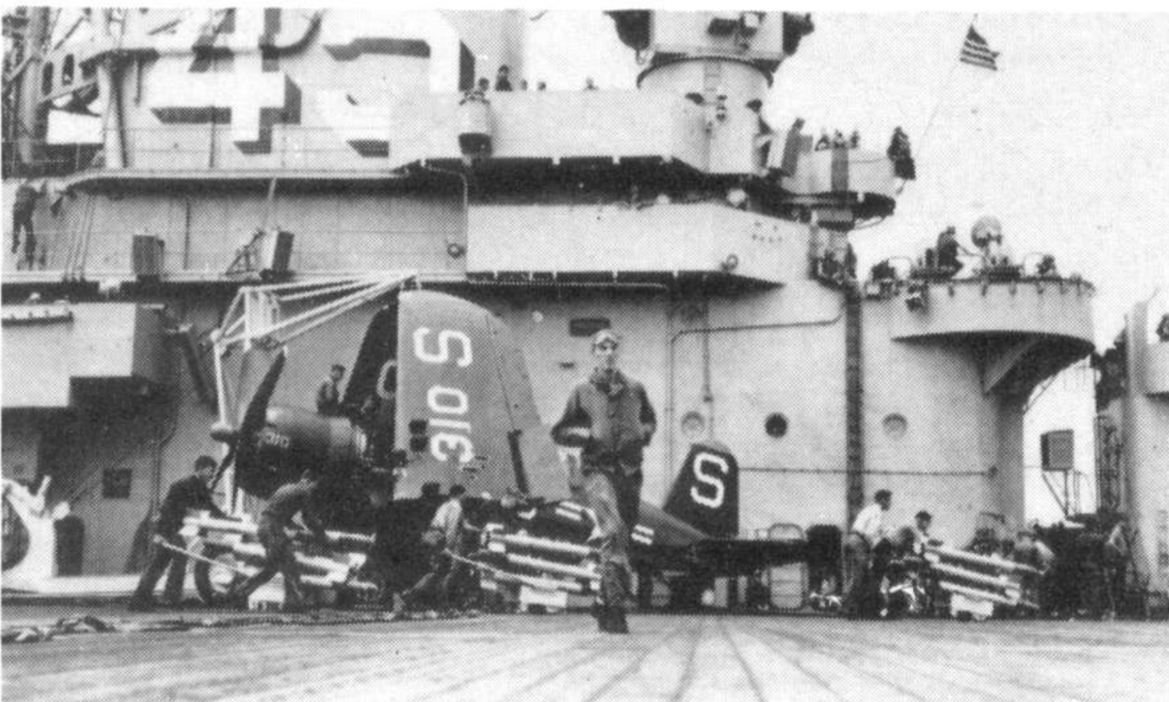
Typical scene aboard a U.S. Navy carrier during Korean War operations; an F4U-4B being re-armed for a ground strike on Communist positions from the U.S.S. Valley Forge. The tail letter "S" identifies CVG-5, and the red tip indicates the third squadron in the Group.
