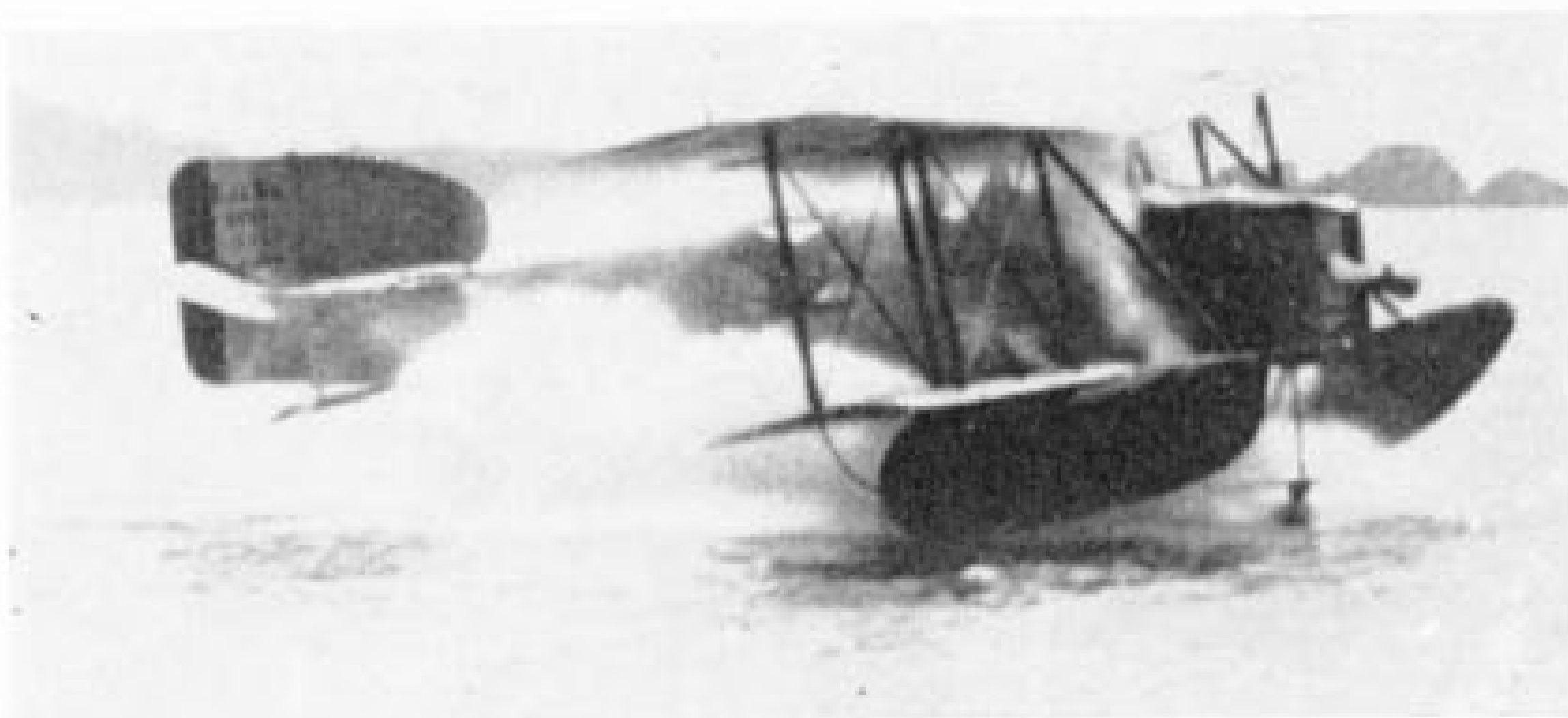
Breguet 14B2 fitted with flotation gear. The aircraft has horn-balanced ailerons, wire trailing edges, the late 14B2 lower wing and underwing skids. (Photos: Jean Noël)
