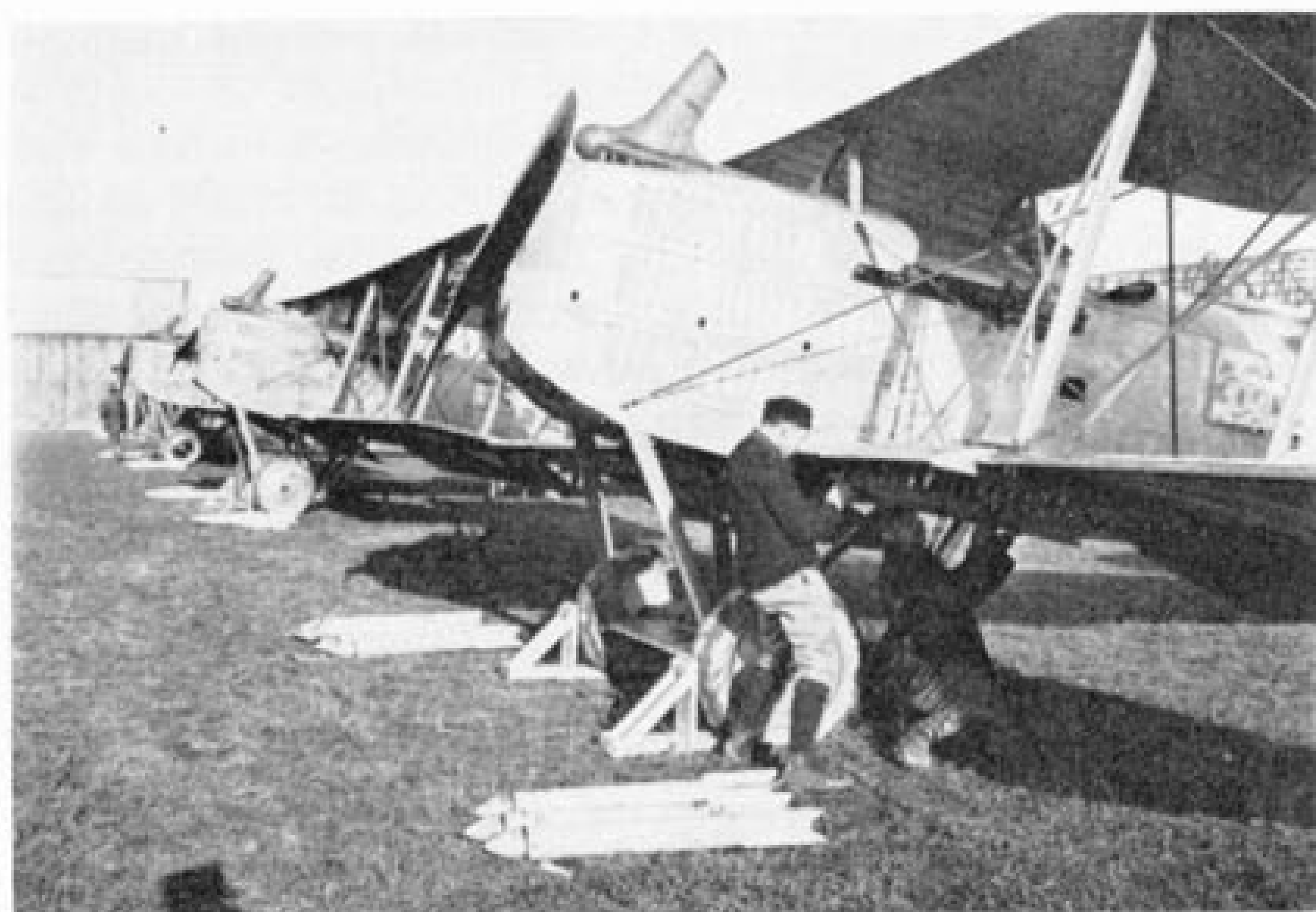
Bombing up Breguet 14B2s of the famous Escadrille BR 66. On these aircraft the fuselage windows are immediately below the upper longeron (this became the standard position), and the gun mounting on the rear cockpit of the nearest aircraft is a T.O.3. (Photo: Musée de l'Air Moreau 1730)
