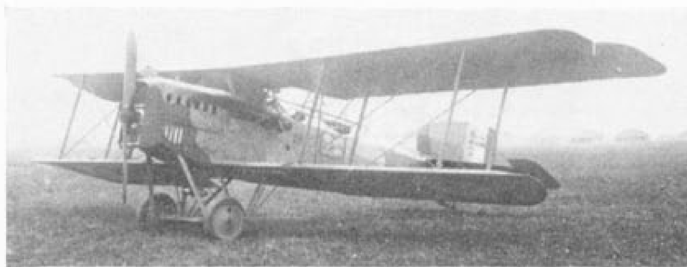
Breguet 14B2 No. 4360 with Liberty 12 engine. This aircraft is remarkable for having the projecting wing portions on the lower wings combined with the late 14B2 wing structure, in which there were no flaps on the lower wings. The revised plan-form of the lower wing tips can be seen and should be compared with that of No. 670 on page 5. As explained in the text, this revised wing arrangement was fitted to Breguet 14B2s that had the horn-balanced ailerons; this aircraft also has wire trailing edges. (Photo: Jean Noël)
