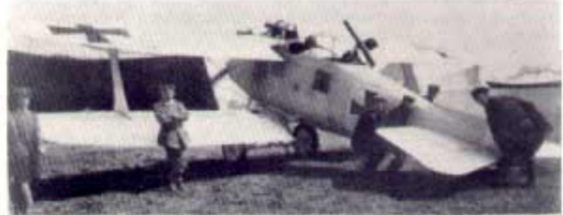
Left: Some C.II's were fitted with a wire gun deflector between the cockpits, to prevent the observer accidentally cracking the pilot's skull or shooting his ear off in the heat of combat. Right: The first major external modification was to mount a fixed forward-firing MG 08/15 Spandau machine gun; this necessitated a redesigned square crash pylon.
