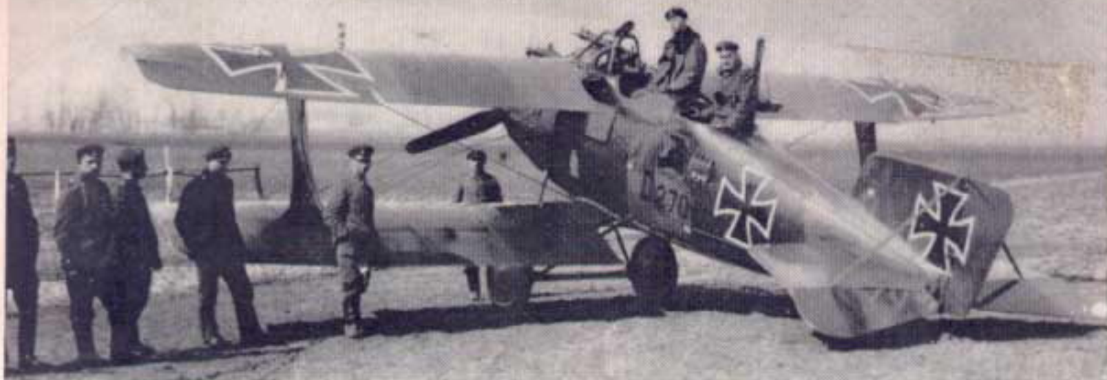
A fine study of Roland C.II 2701/16 with enlarged fin and rudder. This last modification was an attempt to eliminate side-slipping and spinning tendencies. (Photo: A. Imrie)
