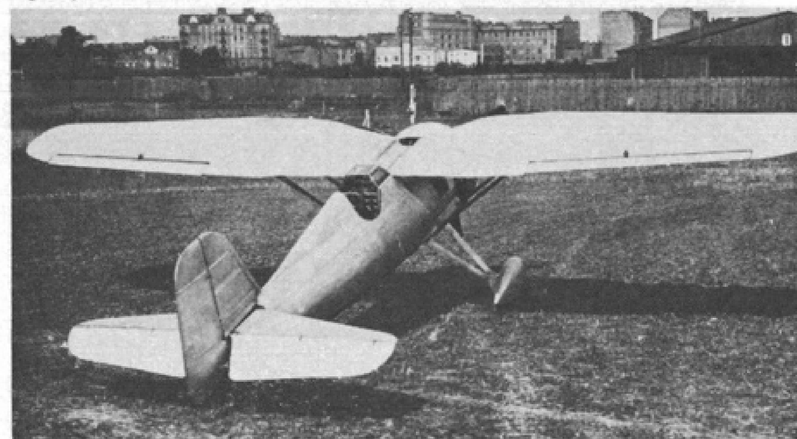
The P.24/II, Super P.24, which established an International Speed Record for radial-engined fighters at 414 km./h. (257.2 m.p.h.).
