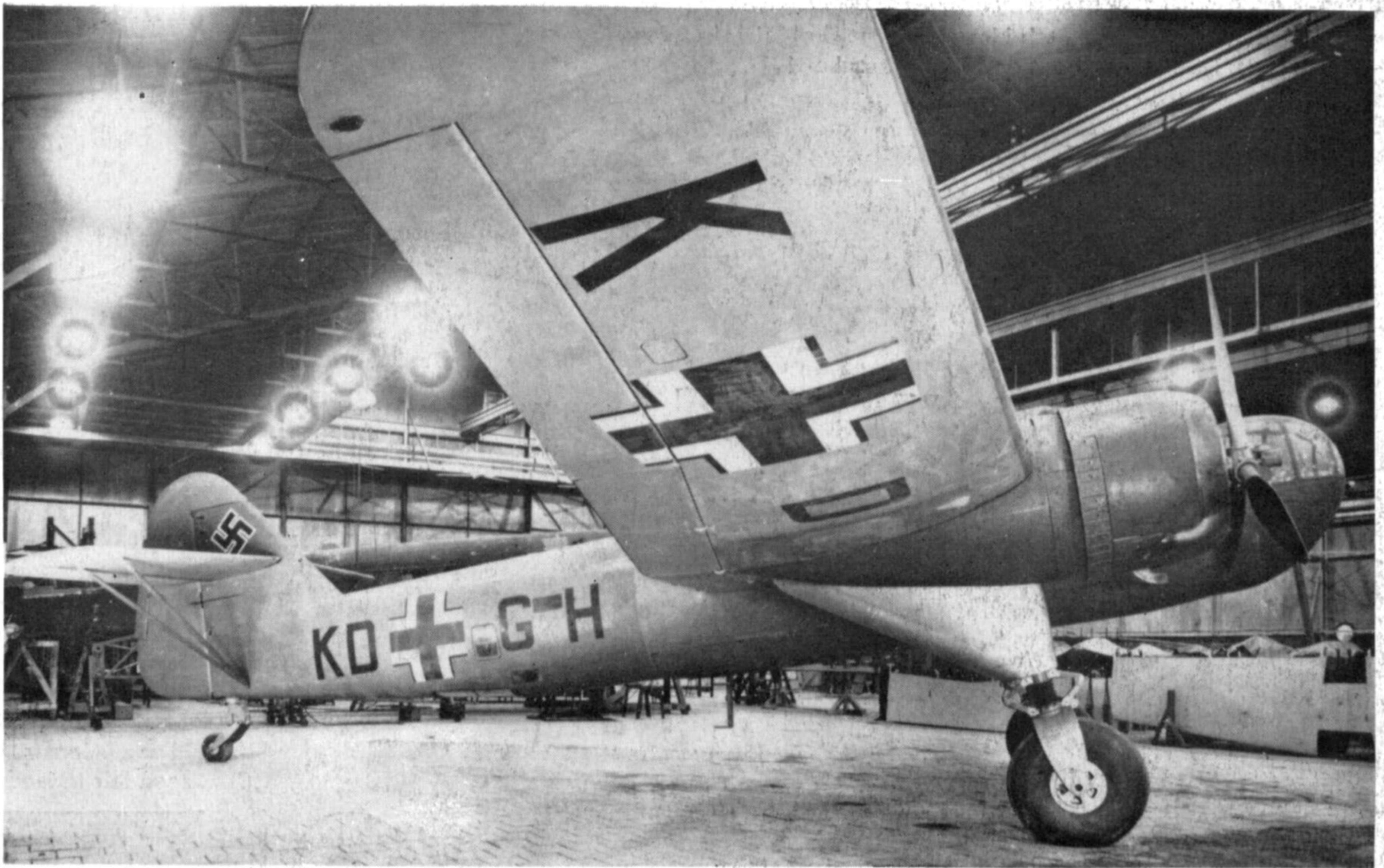
Two views of the sole T.VIII-L ordered by Finland but taken over by the Germans. Note the fixed undercarriage and, in the lower view, the bomb-doors.
