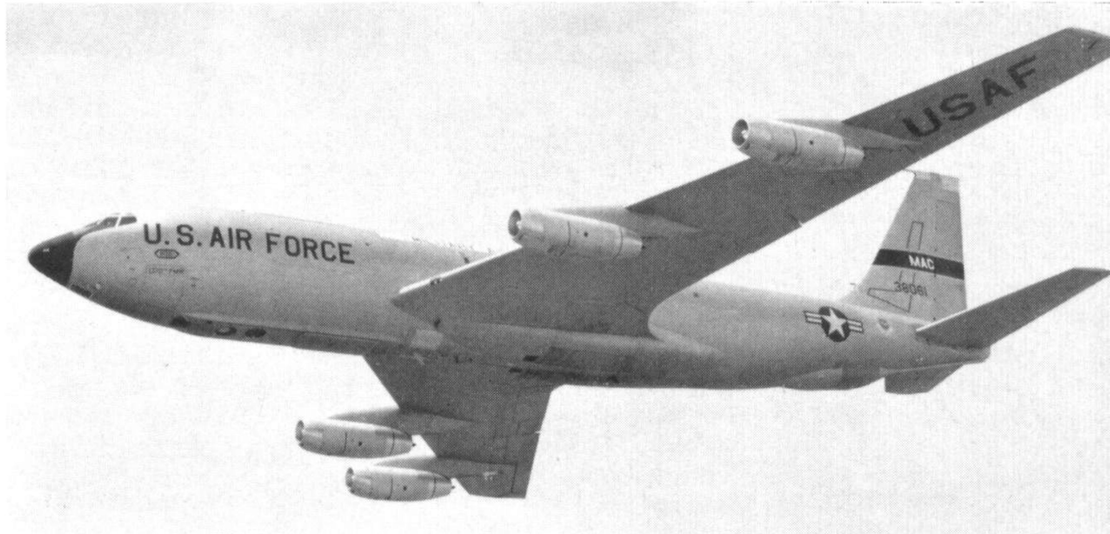
(Above) Modified still further with a twenty-wheel rough field landing gear, the "Dash Eighty" made a series of landings and take-offs from the untreated sand and mud surface of Harper Dry Lake, California.
