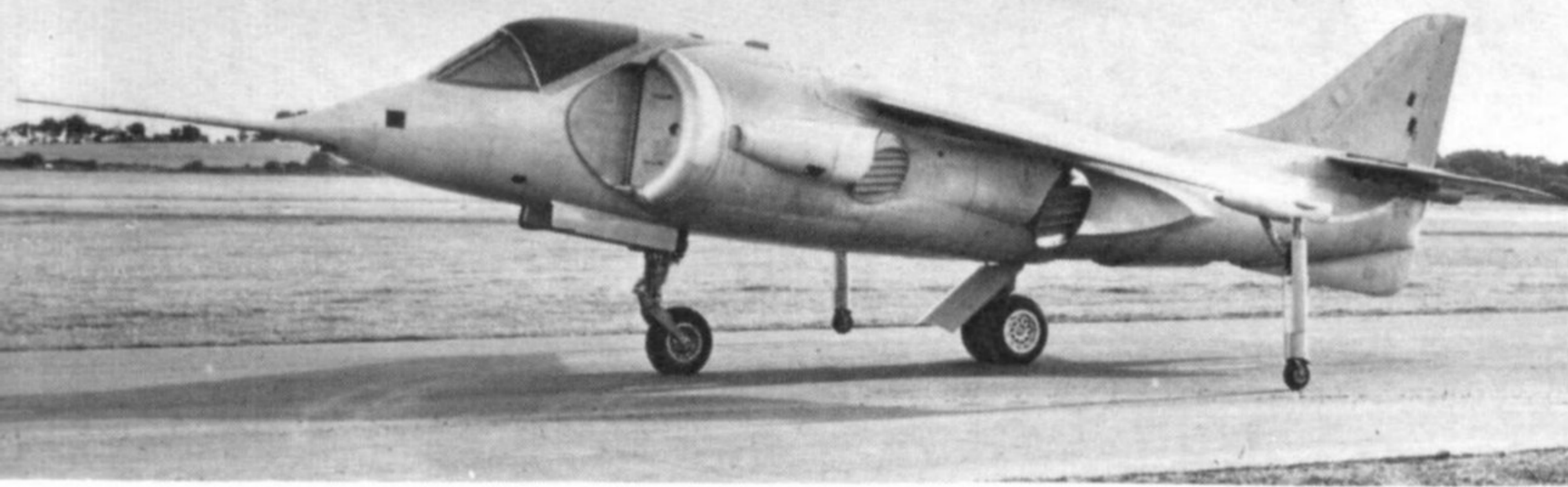
Roll-out picture of the first prototype P.1127, XP831, taken on 17th August 1960. The cockpit canopy is still protected by masking material and various minor panels are not fitted. (Neg. No. EXP255/60)
