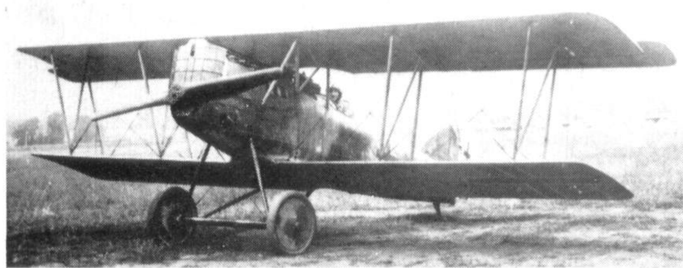
D.XII 2690/18 captured and tested by the French; and (below) 2670/18 flown as war booty in Canada by de Plessier of No. 1 Squadron, Canadian Air Force. Note the shorter, thicker undercarriage as compared to earlier production models.
