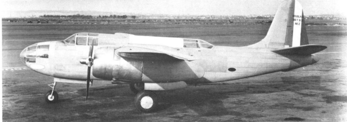
The second DB-7 of the French batch; the tail lettering DB-7 B-3 indicates "DB-7, three-seat bomber." (Photo via the author)
