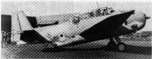
The second XTBM-3 prototype (Bureau of Aeronautics number 2545), which made its first flight on December 20, 1942. This aircraft differed mainly from the first prototype in having a large dorsal fin, a feature retained for all production aircraft.
