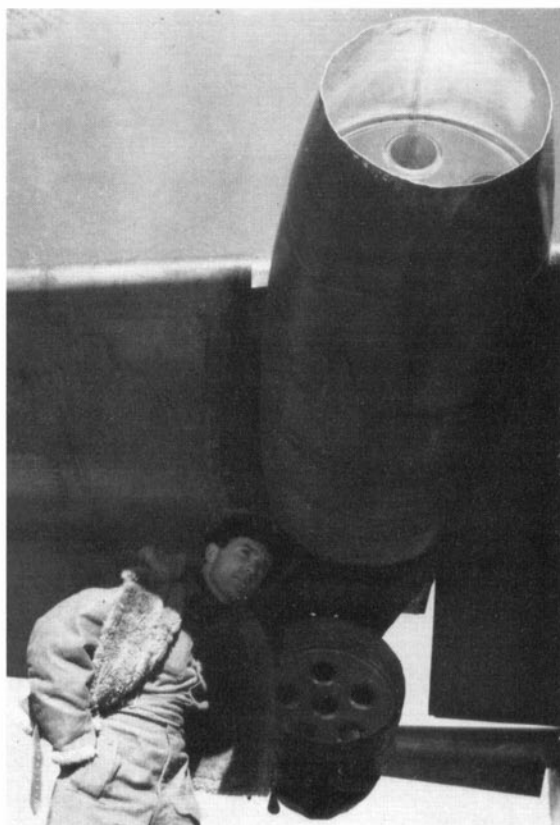
Prior to evacuating Rheine airfield, the Germans removed the underslung Jumo 004 B motors from W.Nr. 140349, a burnt-out Ar 234 B, and substituted dummy motors. Here, an R.A.F. officer examines the substitutes. Although incapable of deceiving a close observer, it is possible that these false "engines" would not have been spotted by Allied photo-interpreters poring over cover of Rheine brought back by high-flying reconnaissance aircraft. (Photo: Imperial War Museum ref. CL 2415)
