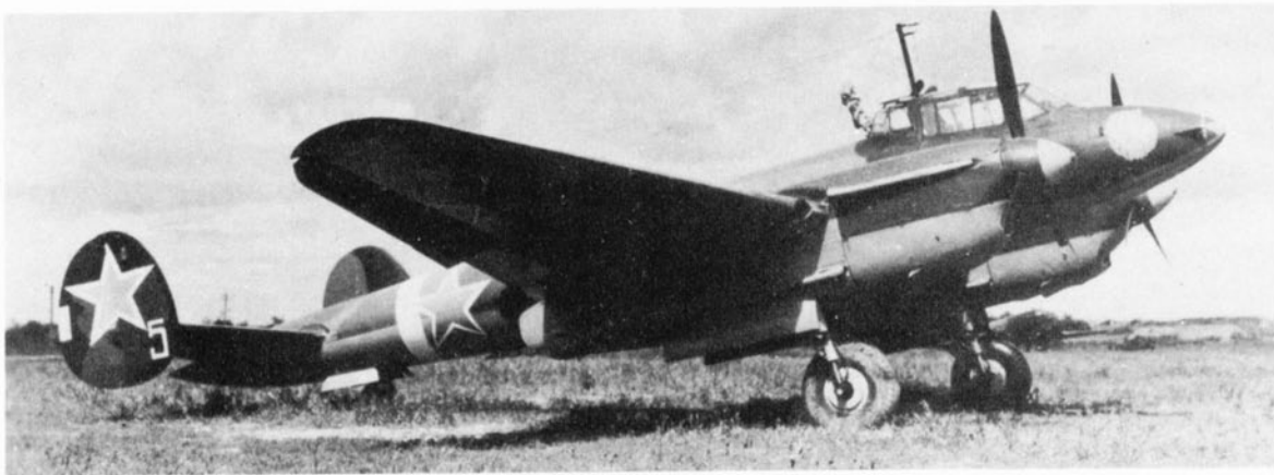
An excellent photograph of an intermediate production Pe-2 with more rounded propeller spinners and the original FT dorsal turret. This is the subject of a colour side view on page 124. (Photo: Airphotos, Jamestown, N.Y., U.S.A., ref. 1955)
