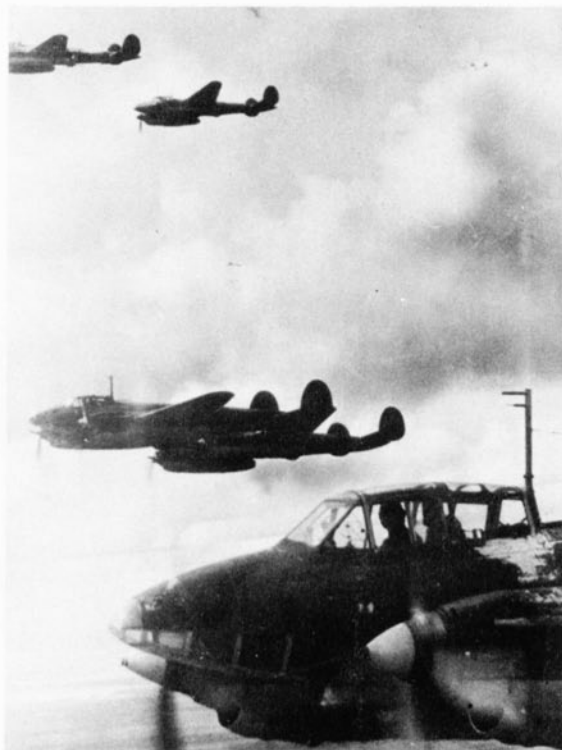
Early production Pe-2s, Winter 1941–2. Middle Pe-2s lack spinners. The dark shape behind the pilot in foreground Pe-2 is his extensive head and back armour protection.
