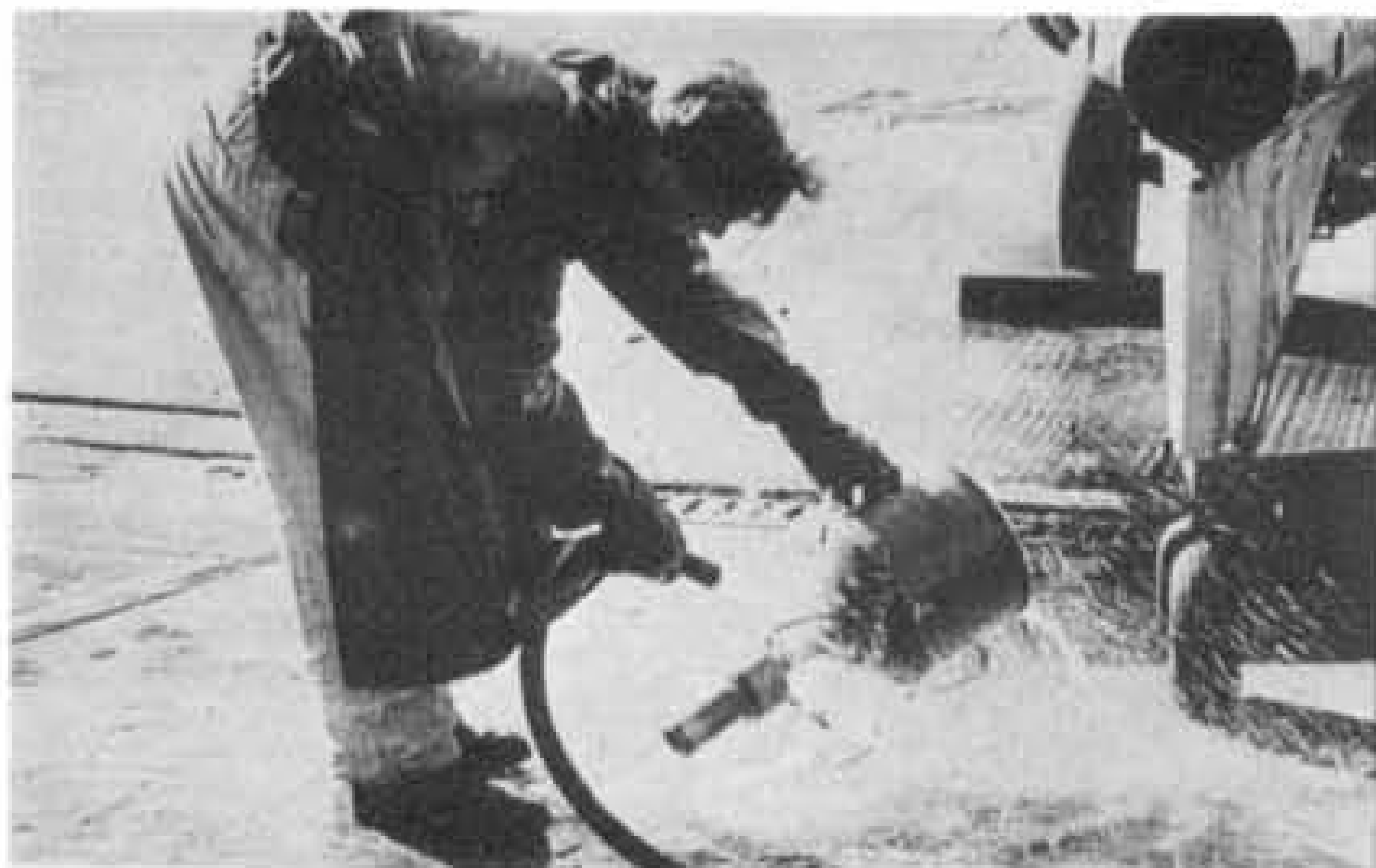
Wearing an acid-proof smock, a Luftwaffe mechanic hoses out the 'Trichter' or special funnel used in transferring the Komet's C- and T-Stoff from the bowser to the aircraft's tanks. Absolute cleanliness was essential to prevent accidental explosions.
