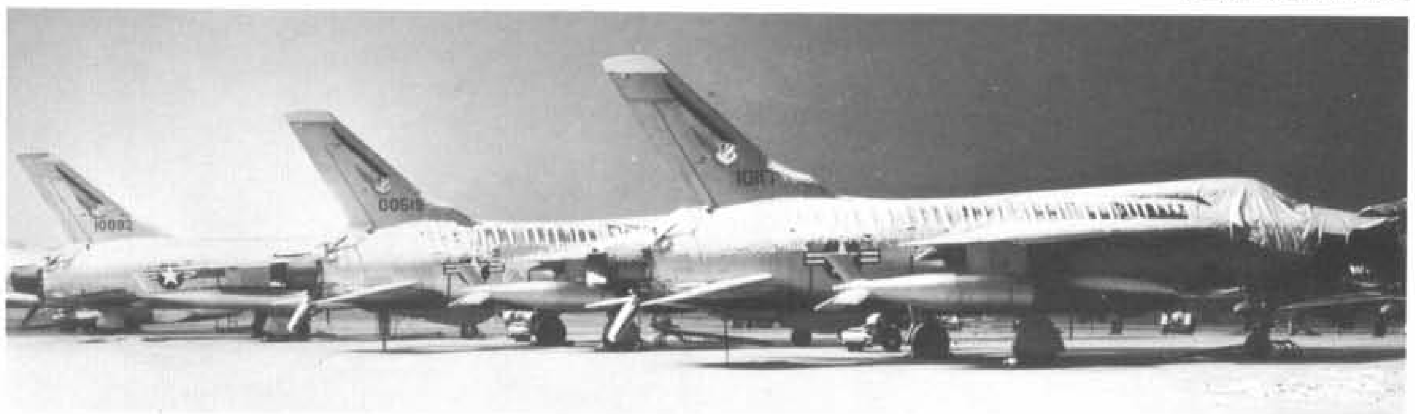
Only poets and skiers appreciate "the mantle of snow"! Winter 1963, at the 49th Tactical Fighter Wing's European base, Spangdahlem AB, West Germany. The original policy of open-air deployment revealed sealing and corrosion deficiencies resulting in "Operation Look-alike" whereby earlier F-105Ds (D-10s, -15s & -20s) were suitably modified to F-105D-25RE standard at Brookley AFB, Mobile, Alabama. Externally, the most obvious change was from natural metal finish to a protective acrylic aluminiumized coating overall. The F-105Ds have been treated at Mobile although serials show they were built as (left to right) an F-105D-15RE (61-0092), an F-105D-10RE (60-0519) and an F-105D-20RE (61-0117).
