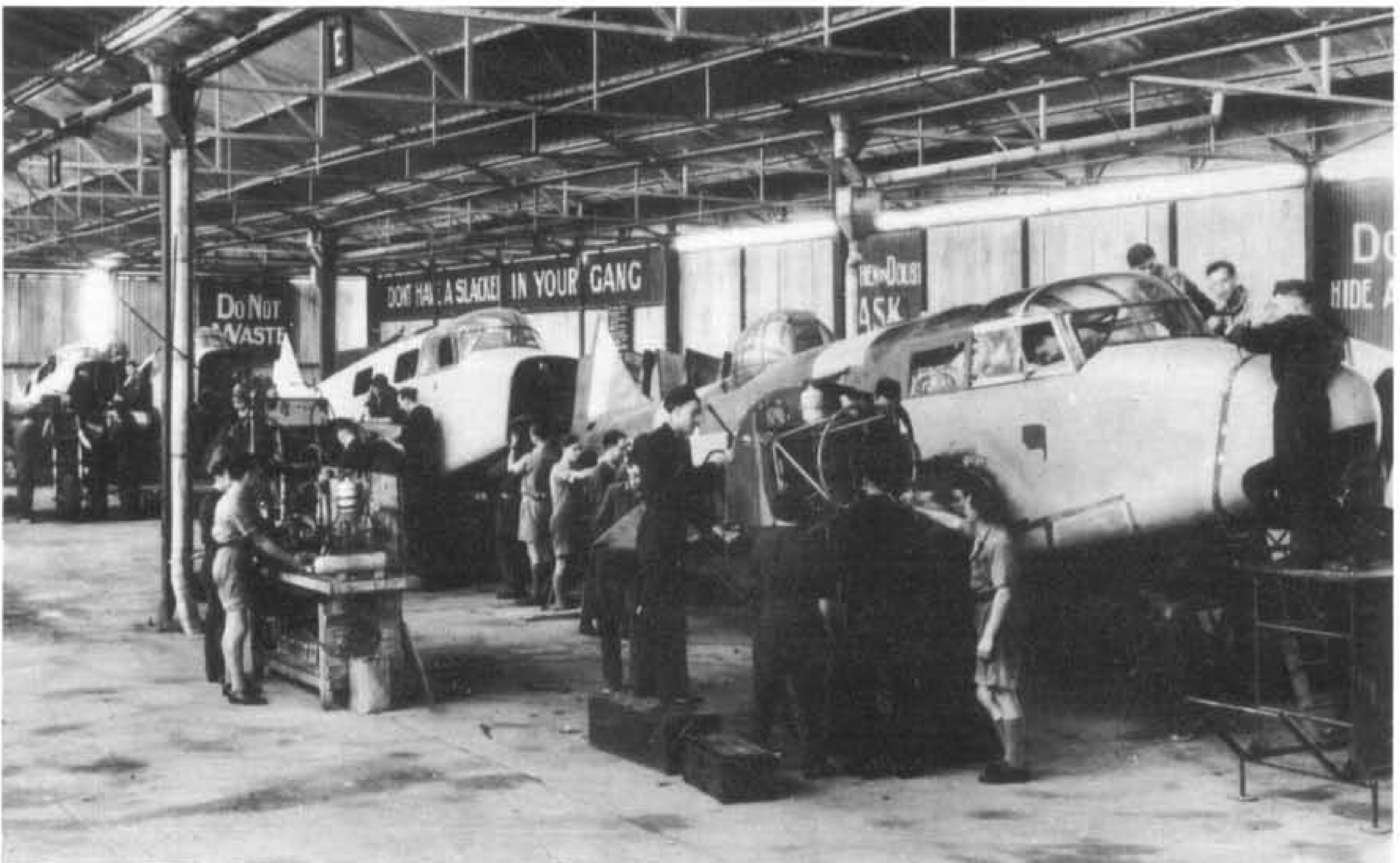
Airspeed Oxford Is being assembled in Rhodesia during the War for the Empire Air Training Scheme.
