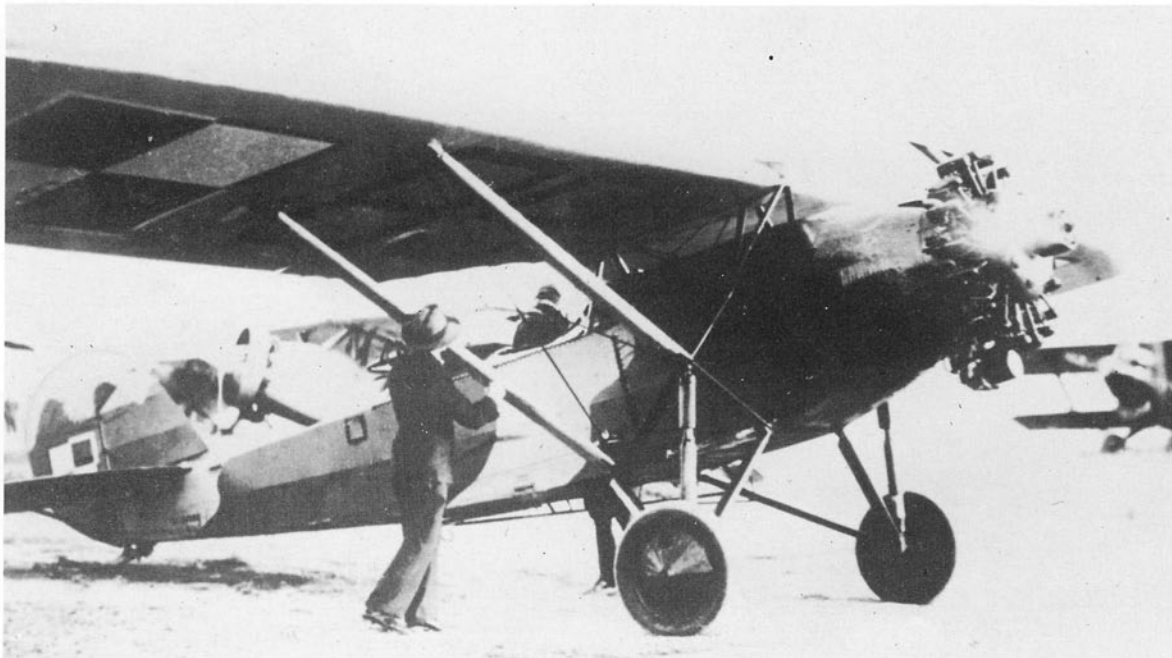
An early production R-XIIIA liaison/observation monoplane, finished in burnt umber, green and yellow ocher camouflage, with light-blue undersurfaces. (Photo: A. Glass)
