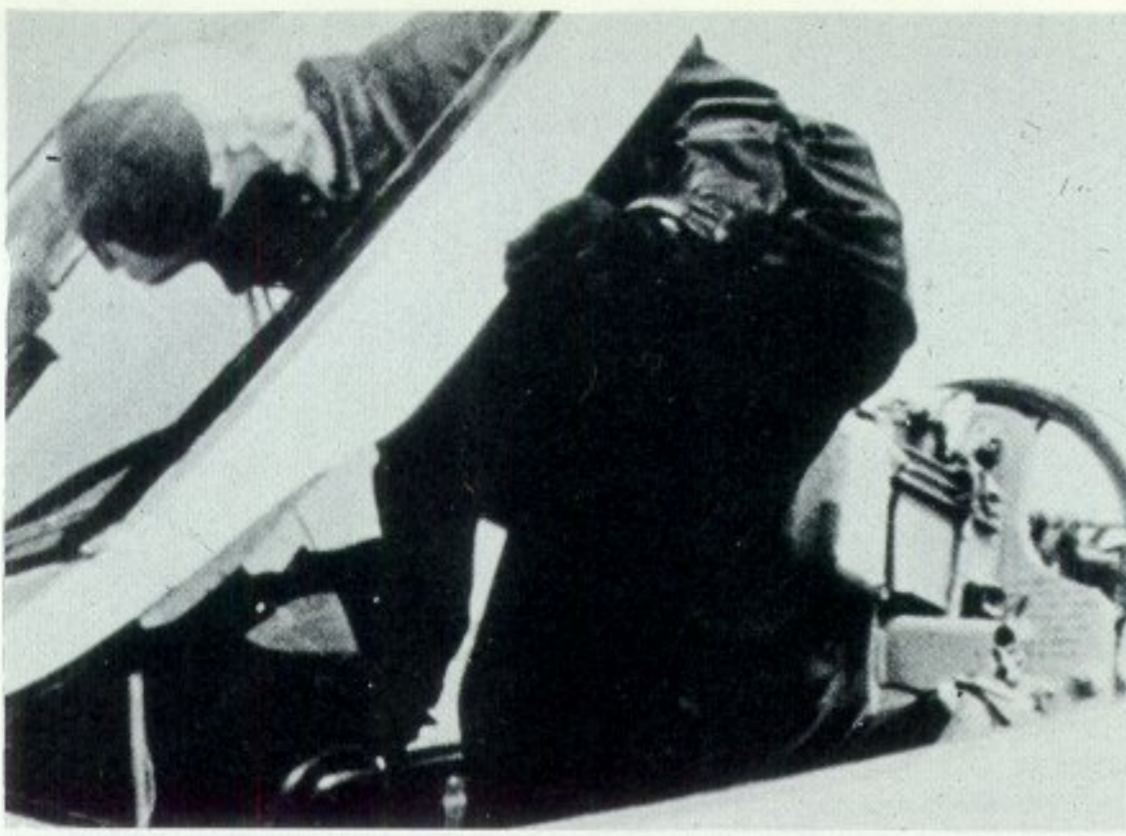
All the initial production series of the single-seat MiG-21 featured a cockpit canopy arrangement unusual in that it hinged about the base of the armoured windscreen. These 1962-period views show a Soviet pilot climbing aboard and being enclosed by the canopy. Additionally, if the pilot had to eject, the canopy separated from the aircraft along with the seat to provide protection to the pilot against buffeting until the ejection-seat was slowed down by its drogue chute. (Photos: "Interavia", Geneva, Switzerland)
