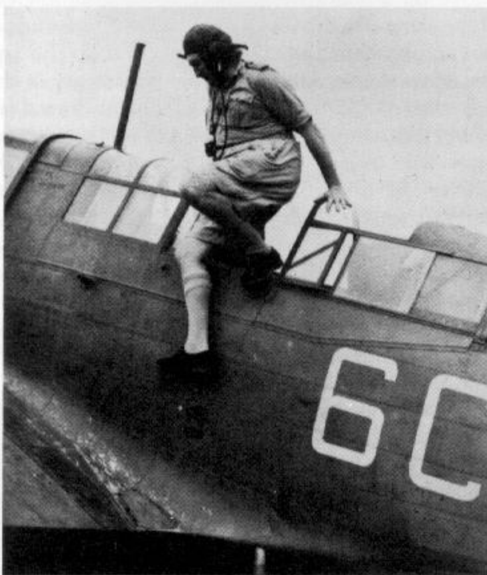
Captain T. Troubridge, RN, commanding Indomitable , climbs out of an 800 Squadron Fulmar II at RAF Port Reitz, Mombasa, after flying ashore from the carrier in June 1942. Note the sliding panels and the braced, hinged panels which gave the Observer an undistorted range of direct vision through which to take compass bearings. (Photo: G. Wallace)
