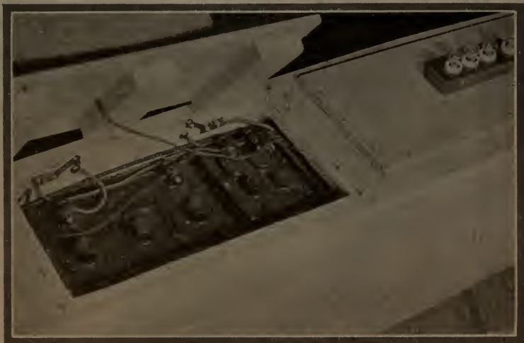
Fig. 231—The central hatch lifted, showing the storage batteries. The signal lamps are shown at the right
