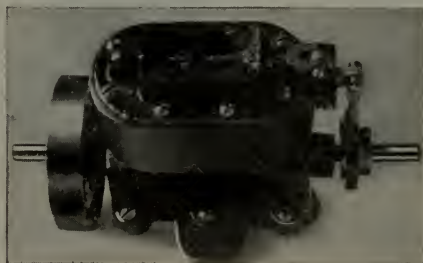
Fig. 99—Top view of the engine showing the steam chest uncovered
