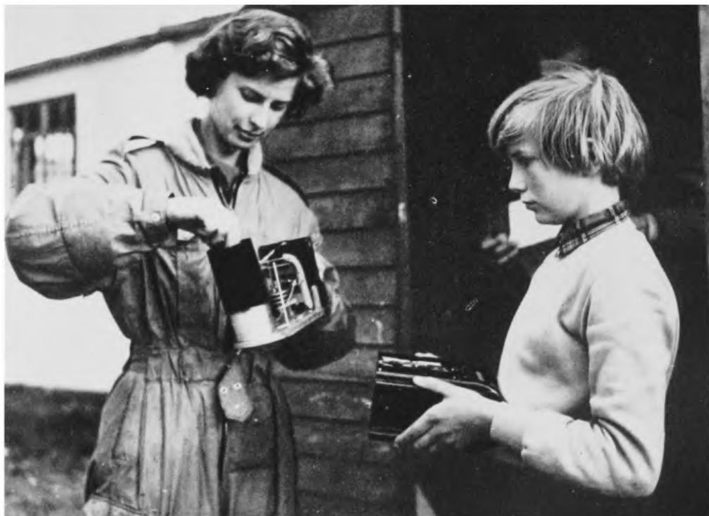
18. (above) In case the opportunity for a record flight occurs the barographs are always sealed, and if the pilot is successful may only be opened by an official observer, because the trace on the drum will be needed as evidence that the record flight took place. Sticky paper is put over the join as a seal.
