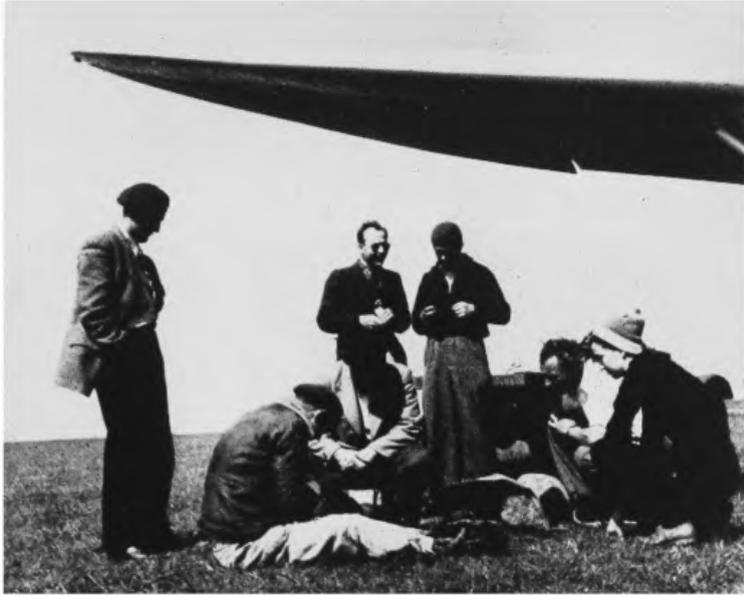
42. Should the launching cable break, it is soon repaired by the members. If it is a stranded steel cable a Fisherman's Knot is normally used and if it is solid wire then a Reef Knot or Whatnot is quick and satisfactory. (see p. 57)
