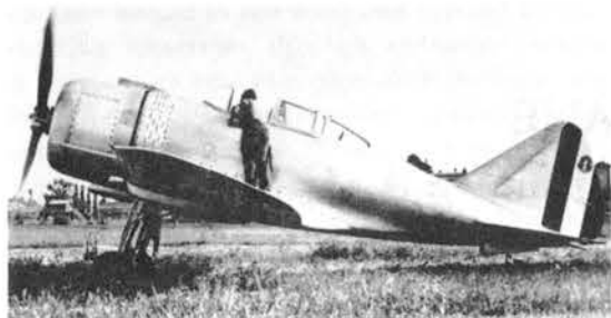
Above left, the prototype Re 2000 in its original form. Right, the same machine after modifications to the carburetor air intake and the addition of a spinner (MM 408)
