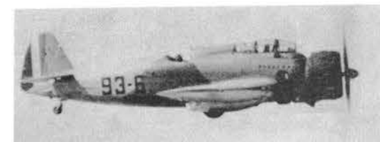
Above, a two-seat Breda 65bis reconnaissance bomber. A flexible machine gun was often fitted.
