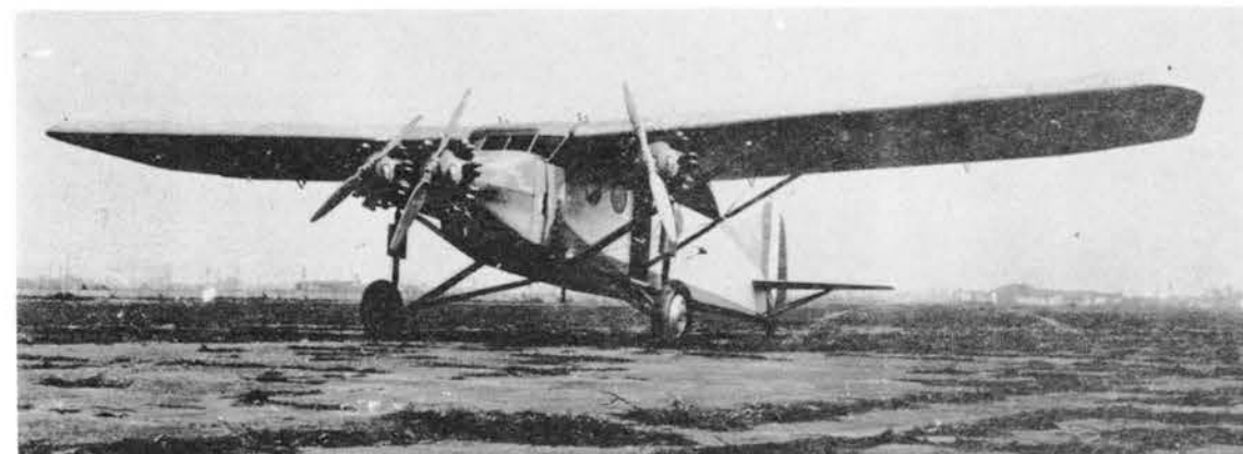
A Ca 101 colonial monoplane fitted with three Alfa Romeo D2 radials.
