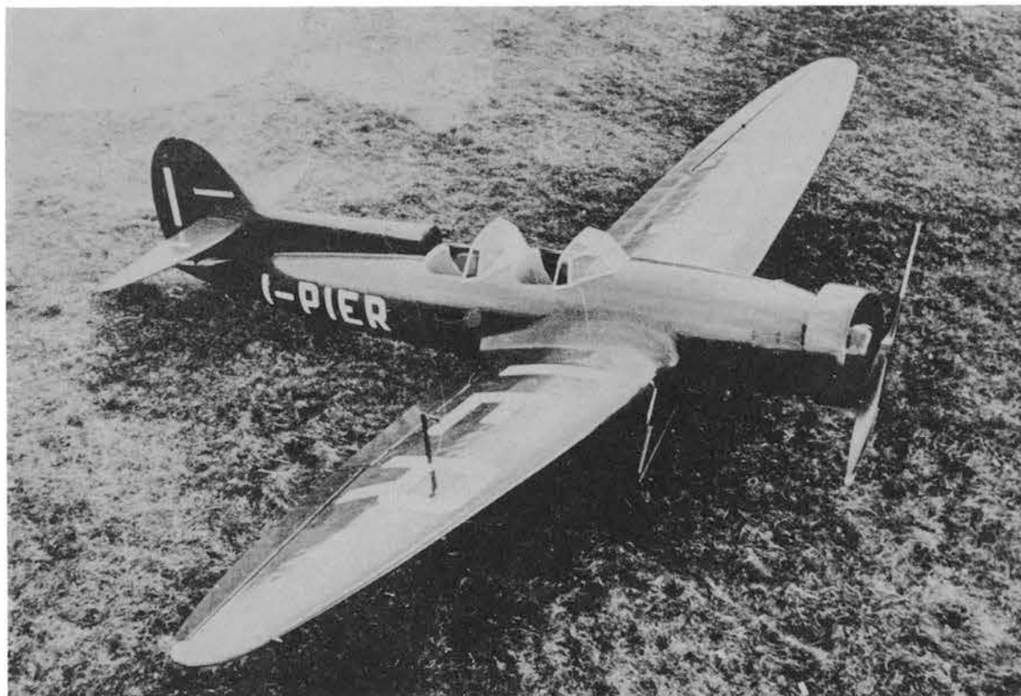
The S.A.I. 3 S, fitted with a German Bramo Sh 14 A4 radial engine and open cockpits. (I-PIER)
