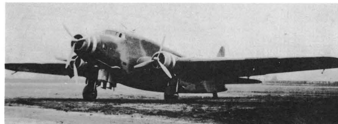
The prototype SM.82 bomber with bombardier position extended. Also visible is dorsal turret.
