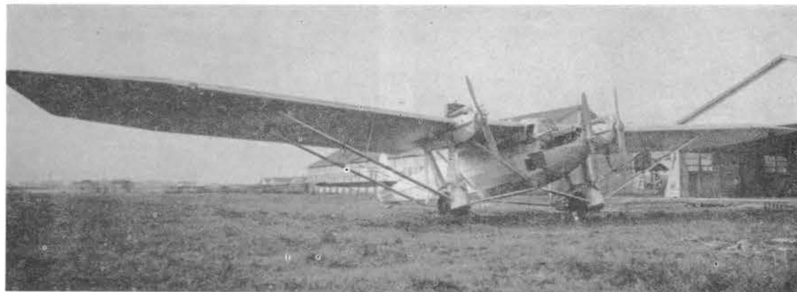
The extremely long wings of the Ca 95 heavy bomber are apparent in this view.
