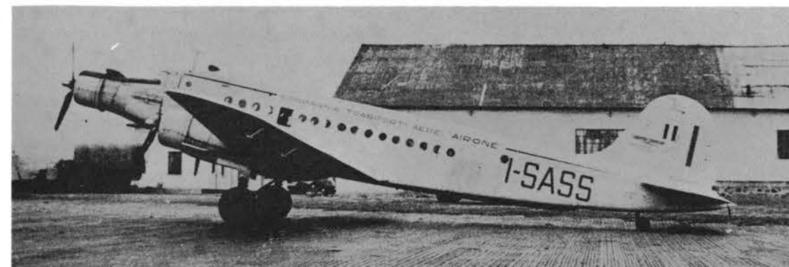
The G.12L was a postwar model for 18-22 passengers. Note longer fuselage, modified fin. (1-SASS)
