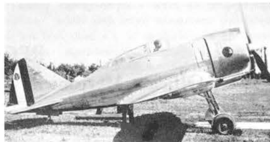
Above left, the prototype Re 2000 in its original form. Right, the same machine after modifications to the carburetor air intake and the addition of a spinner (MM 408)
