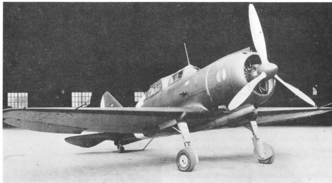
The Re 2003 two-seat reconnaissance bomber with the original Falco-type engine cowling and spinner.
