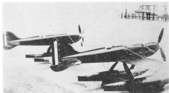
The MC.72 employed the 3100 h.p. twenty-four cylinder AS.6 engine and contra-rotating airscrews.
