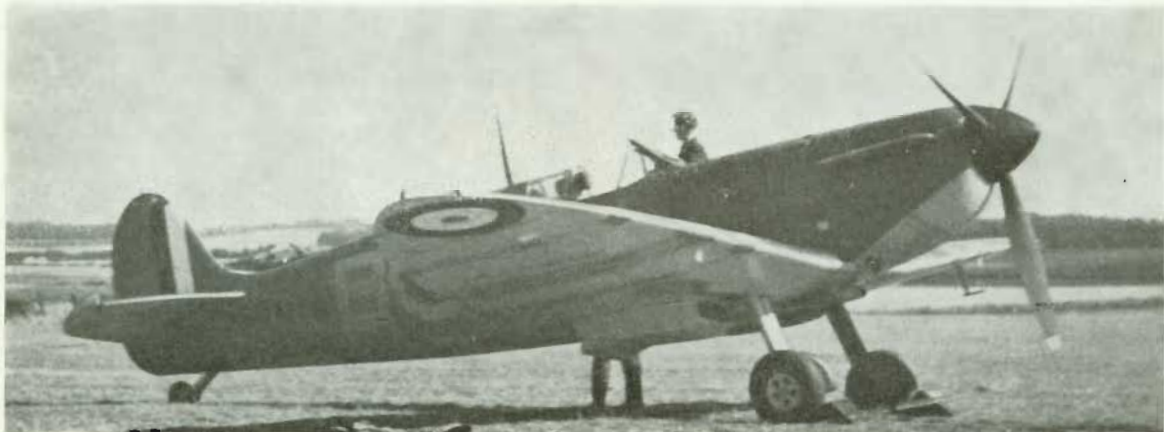
(Above and below) Spitfires of No. 19(F) Squadron. Both aircraft have Dark Green and Dark Earth upper surfaces and Sky under surfaces. The aircraft above has 25in. diameter under wing roundels, while the one below has 40in. roundels. Both aircraft have 7in. wide fin stripes.
