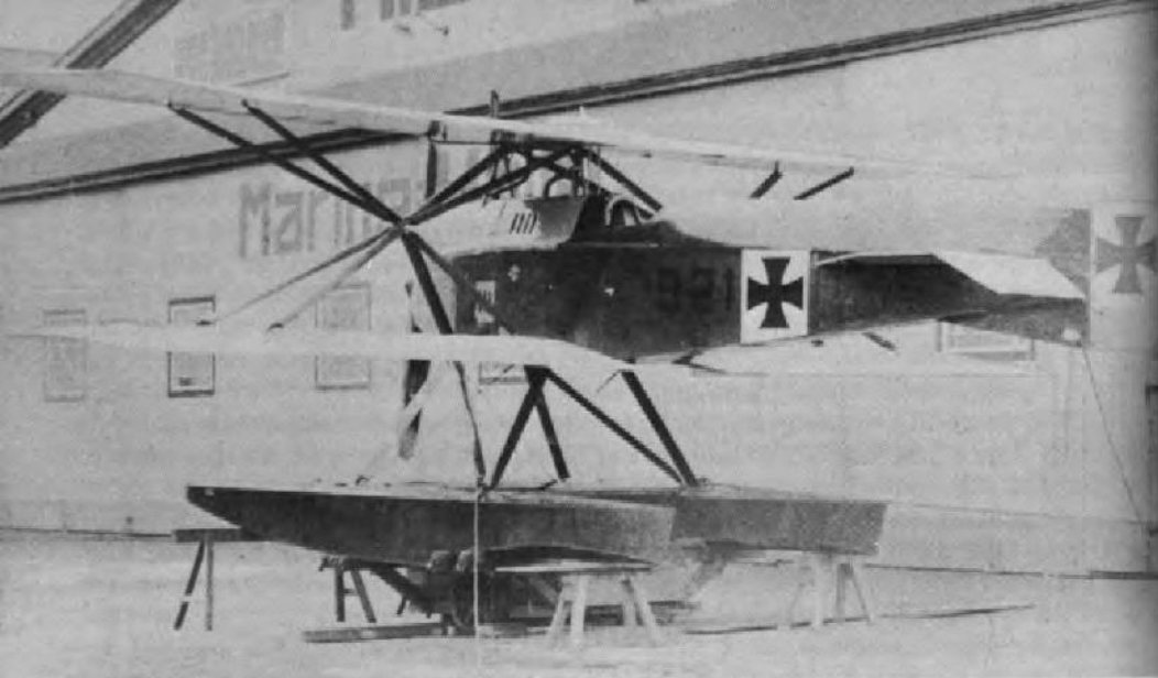
ABOVE: Wooden pontoon floats typical of floatplanes from 1910 to late 1920s. Aircraft here is a Hansa Brandenburg KDW Scout. BELOW: Ultimate development of the wooden pontoon seen here on Blackburn Dar (Civil) in 1924, shows extremely fine workmanship and high gloss finish ('Flight International').
