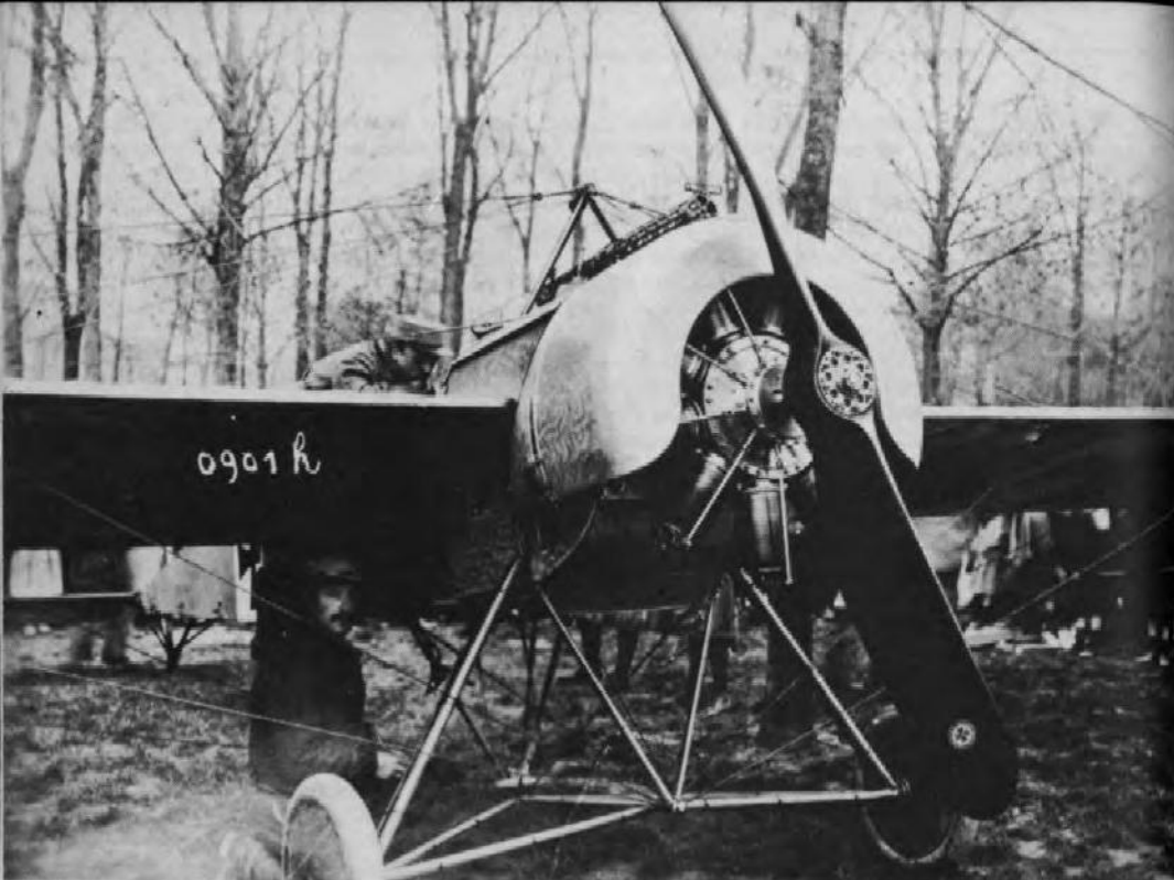
ABOVE: Garuda propeller on a captured Fokker EIII. Note typical 'butter pat' shape of this airscrew used on most of the early Fokkers. The trade mark is a cross patée on a white circular field surrounded by the letters 'Garuda Feldpropeller'. Garudas were made from layers of mahogany.
