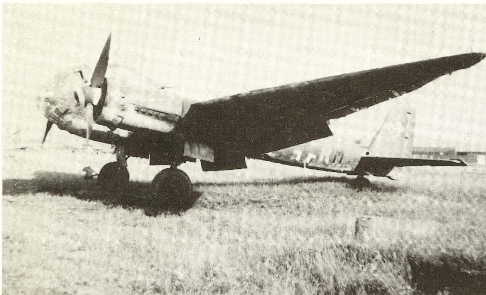
Left: Captured at Kassel, this Junkers Ju 188 A-2 had its 70/71 uppersurfaces densely mottled with a close spray of 76 Light Blue. Undersurfaces were the usual Light Blue 65 while spinners were black with a white spiral. The Junkers VS 11 wooden prop blades were Dark Green 71. Although the unit code is obscured, the individual aircraft letter, R, was red with a white outline followed by a black letter M. This is an instance where the Gruppe color (red) was combined with the Staffel color (white).
