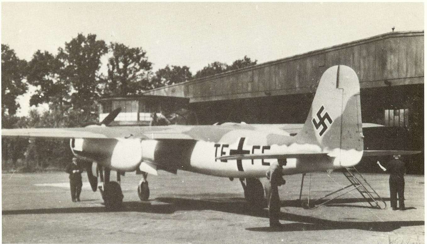
Above: The Focke-Wulf Ta 154 V1, W.Nr. 0001, TE+FE, Kurt Tank's plywood night fighter, is shown here in mid-1943. The camouflage is reputed to have been 02/74/76. Generally, colors 74 and 75 would have been of much lower contrast than we see in this view. Lower: Camouflage for the seventh prototype, the Ta 154 V7, W.Nr. 0007, TE+FK, had been refined to the scheme adopted for full production machines. They employed a base of Light Blue 76, with upper surfaces covered by a random application of Gray-Violet 75 spots. Spinners were Black-Green 70, while the wooden Junkers VS 11 prop blades were Dark Green 71.
