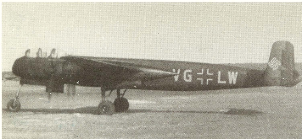
Left: The Heinkel He 219 V3, VG+LW, which flew in late December 1942, is shown here during evaluation early in 1943. Overall finish was Black 22 with registration code letters in Gray 77. Middle Left: Photographed in August 1945, this He 219 A-7, W.Nr. 310 189, formerly D5+CL of 3rd Staffel, I./NJG 3, was camouflaged Light Blue 76 overall including the spinners, with a soft-edge mottle of Gray-Violet 75 over all top surfaces. The small "VI" near the foot step beneath the canopy indicates that the aircraft was fitted with FuG 220d radar with Streuwelle VI (dispersal waveband). Aircraft code letters, D5+CL were most likely Gray-Violet with the exception of "C" which was yellow. Lower: Another He 219 A-7, W.Nr. 190 176, is shown here following capture by Col. Watson's special group at Lechfeld, June 1945. Note this "Uhu" has been victimized and is lacking the lower radar antenna elements and forward windscreen. Minor camouflage variations appear even within the He 219's approved scheme. Note that this example's props and spinners were solid Black-Green 70. The placement of the serial number is also noteworthy.
