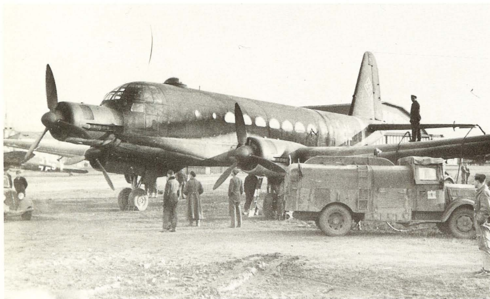
Above: This Ju 52/3m g5e, W.Nr. 7279, 4V+BP (originally TG+ES) was one of a pair which force-landed on January 22, 1945, southwest of Asselborn, Luxembourg. Fitted with flame dampers for night operations, the standard 70/71/65 has been altered by the liberal application of white over uppersurfaces, while the outer portion of the wing's undersurface was in yellow. Reportedly, this machine was on strength with III./TG 2. Left: Logical successor for the Ju 52 would have been the Ju 252, but only 25 were built. This example, Ju 252 V5, DF+BQ, was in 70/71/65, with a yellow tail band. It was operational with LTSt. 290 based at Berlin's Tempelhof airfield early in 1943. All 25 examples of the "Herkules" were considered prototypes being retained for special missions and VIP transports. Below: This Ju 352 A-1, N1+CX, originally attached to Grossraumtransp. st. based at Tutow, was captured after the war and used by the RAF for various ferry missions as AM 18. Camouflage was 70/71/65.
