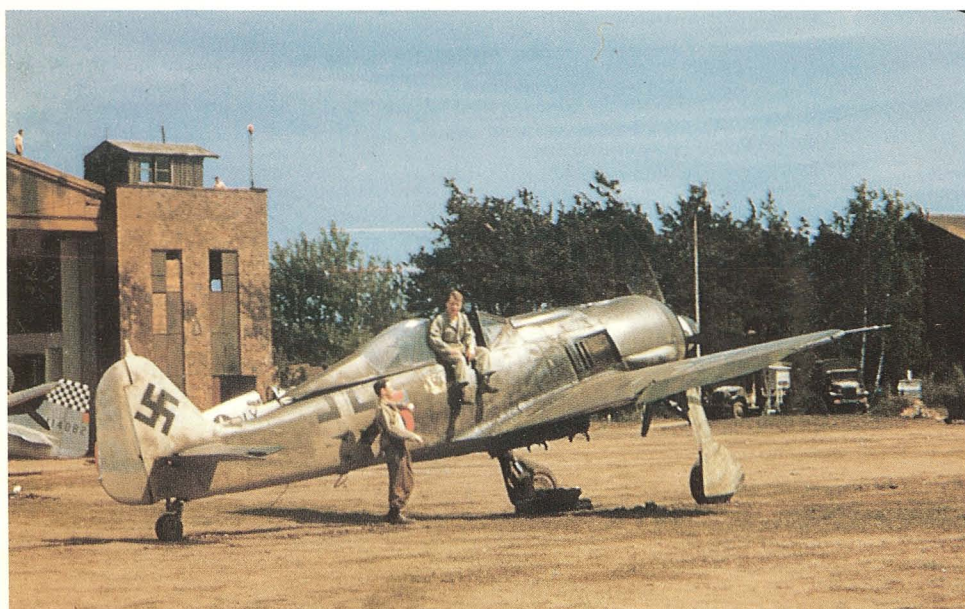
Above: Newly completed Focke-Wulf Fw 190 A-9s at Ago's Oschersleben facility. The entire uppersurfaces were painted Gray-Violet 75 with fuselage undersurfaces and side portions in Light Blue 76. A soft mottle of Brown-Violet 81 and Dark Green 82 was carried along the length of the fuselage. Like the Fw 190 D-9 shown at the top of page 38, the rudders were Light Blue 65 mottled with 75. Note that the color of the undercarriage covers (and presumably the wing undersurface) is nearly identical to the "Sky Gray" shown on page 41. Left: Although camouflage of this Fw 190 A-9, "Red 5", is similar to the ones above, the fuselage sides appear to be RLM Gray 02. Bottom: A high magnification photographic blow-up reveals a near perfect Fw 190 D-9 (right) once operated by the 2nd Squadron's Technical Officer. Uppersurface are 82/75/76 with a mottle of 82. Although not distinct in this blow-up, the remains of a Bf 109 K-4 may be seen to the lower left undeniably camouflaged in colors 75/82/76 with a narrow yellow tail band.
