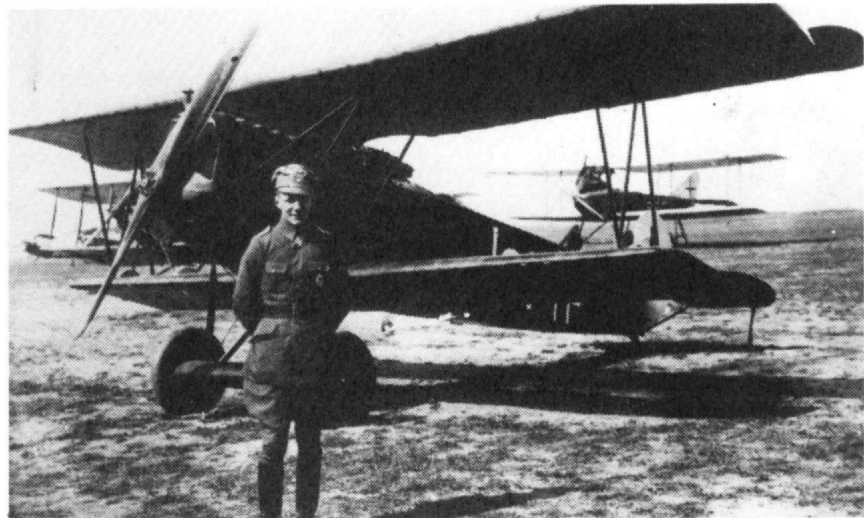
of the aircraft were powered by the Mercedes D.III engine, rated at 160 hp; however, later models were fitted with Daimler and B.M.W. engines for high altitude.
