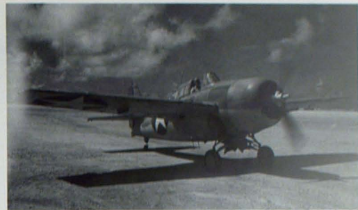
Right: The application of the aircraft number on the forward edge of the cowl or landing gear doors, as on this Wildcat, was an optional aid to the plane captain in identifying his aircraft as it taxied in. Bottom: A SNJ instrument trainer at NAS Melbourne, Florida.
