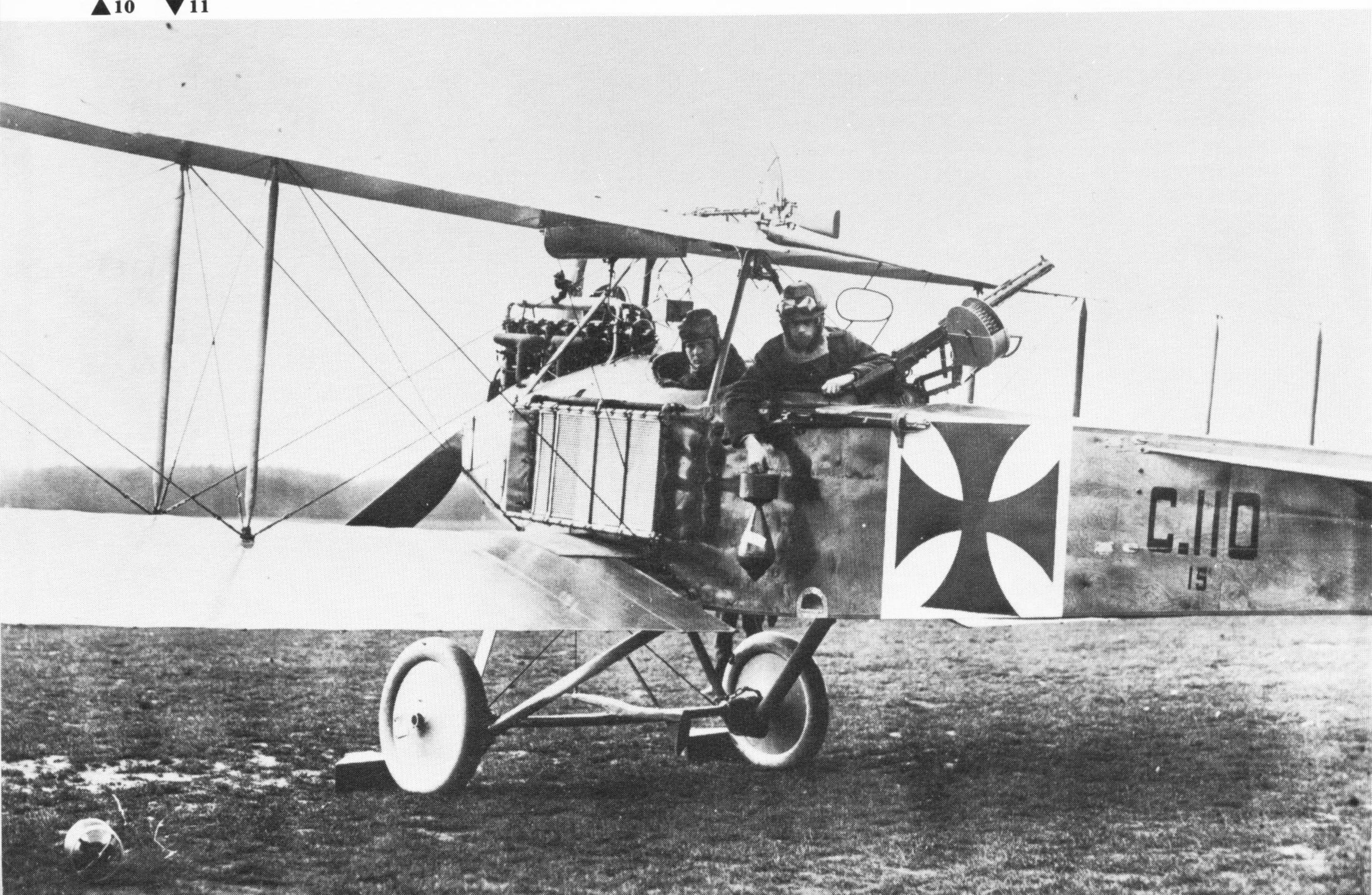
Parabellum LMG 14 on the pivot of the rotatable gun ring, this aircraft carries a Madsen (known as 'Die Muskete' in the service) firing forward over the tips of the propeller, and for good measure a '98 Carabine is strapped to the side of the fuselage. The claw brake pivoted on the centre of the undercarriage spreader bar was a standard fitting on all two-seaters.
