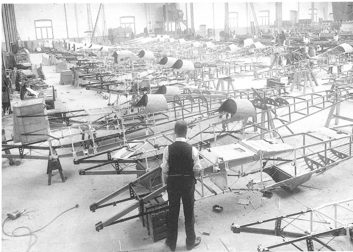
BE2cs under construction at the Daimler Works.
