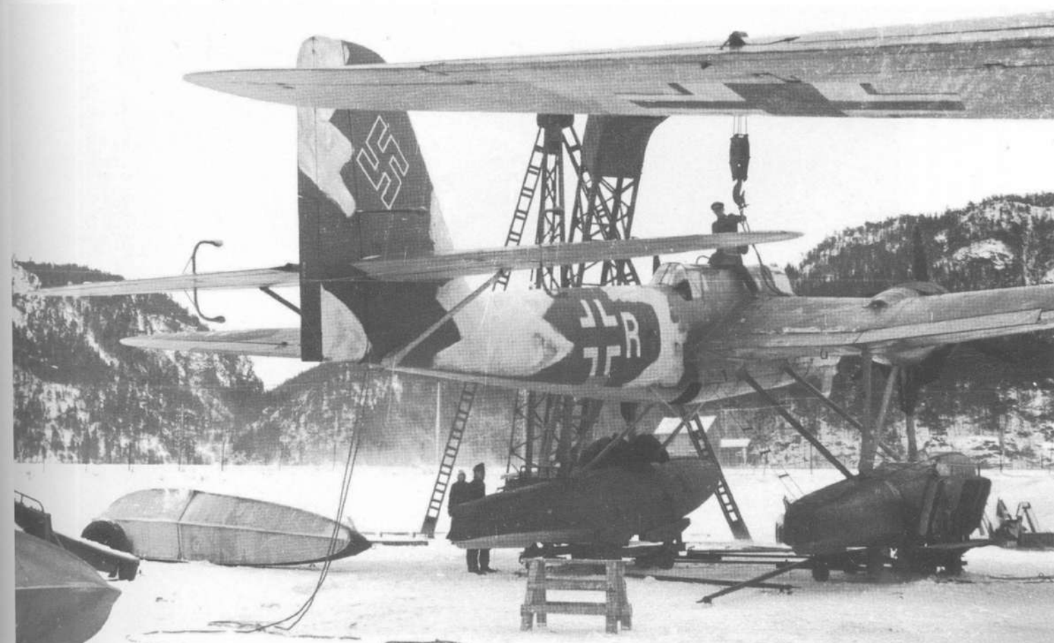
Wearing a partial temporary white finish over its standard 72 & 73 camouflaged upper surfaces, K6+RH, a Heinkel He 115 C-1 of the 1./KFlGr.406 is seen undergoing a float replacement at Trondheim during the winter of 1942.
