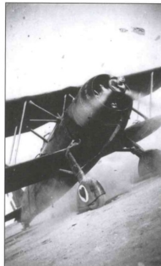
A CR.42 of 77 a Squadriglia , 13° Gruppo has its engine run up at Tripoli Castel Benito, in Libya, during the summer of 1940. Note that the aircraft lacks a spinner, indicating that this photograph was taken while the fighter was being tested following maintenance. The Squadriglia's official badge – a red heart in a white disc – can be seen on the wheel spat. 13° Gruppo (77 a , 78 a and 82 a Squadriglie ) was commanded by Maggiore Secondo Revetria and based at Tripoli Castel Benito airfield when the war started, the unit being equipped with 25 combat-ready CR.42s and 11 CR.32s. It was the only gruppo in Libya to operate CR.42s at this time (Roberto Gentili)
