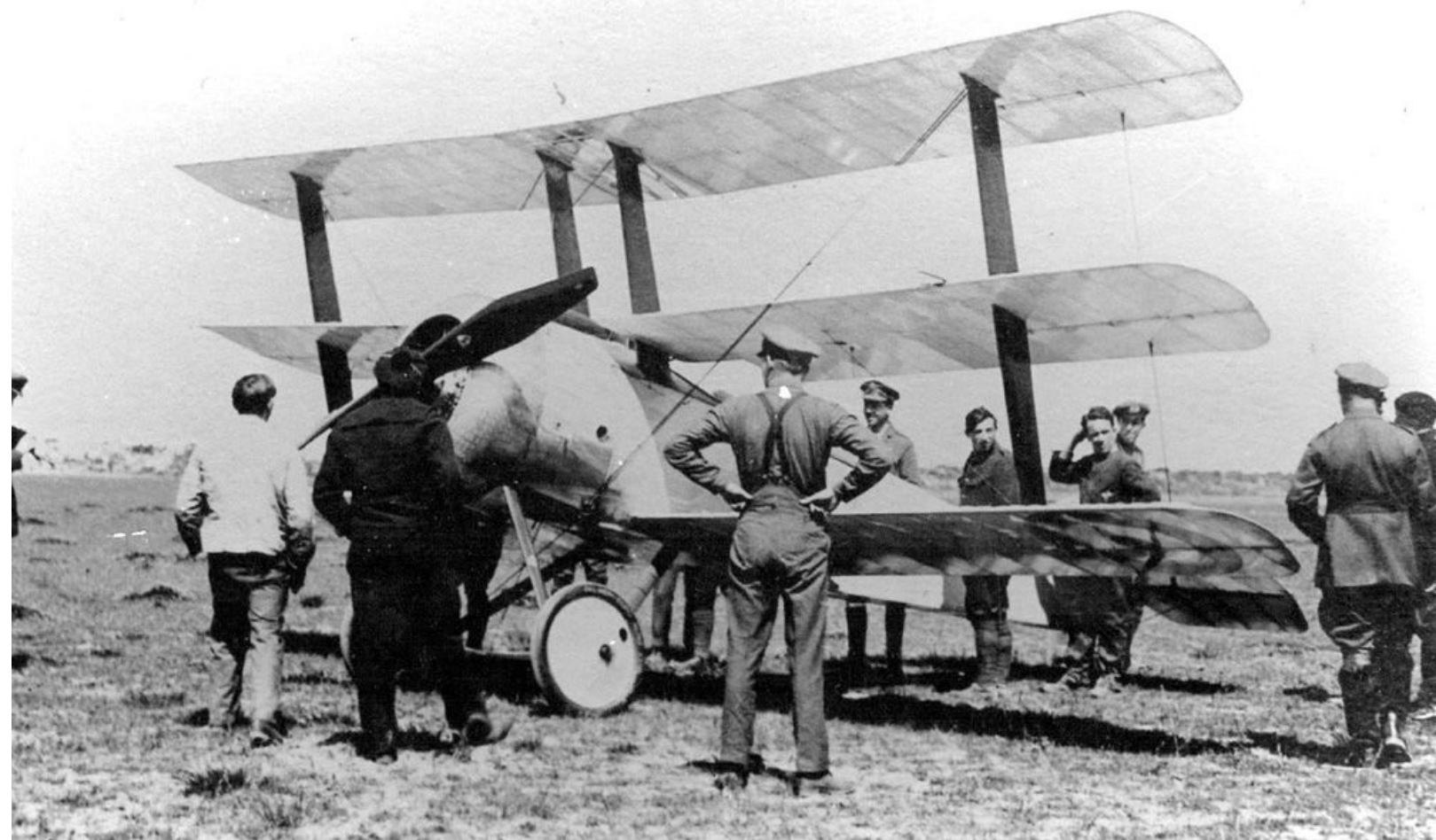
The Sopwith Triplane. This is N500, the prototype machine, which was flown and tested by Captain R. S. Dallas. This uncamouflaged machine is seen after its arrival at St Pol in June 1916. Triplanes served in several RNAS squadrons during 1917,
