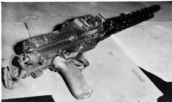
The MG 81Z (Zwilling-Twin) machine gun, standard late model defensive armament. (Photo: J. L. E. Maskall)
