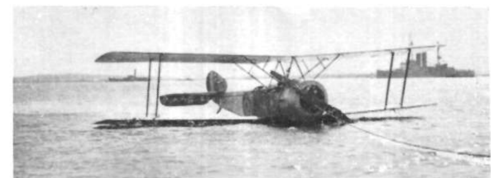
9390 photographed at the Isle of Grain on 8th September 1917, fitted with biplane hydrovane, inflatable air bags mounted on boards that were braced to the upper longerons, and auxiliary bracing at the mid points of the outboard cabane struts.
