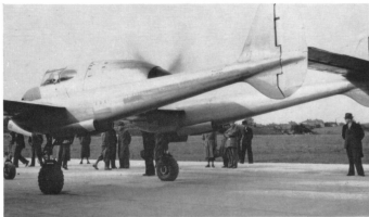
The initial prototype of the J 21A series, serial number 21001, first flown 30th July 1943. Note the original form of the tailplane.
