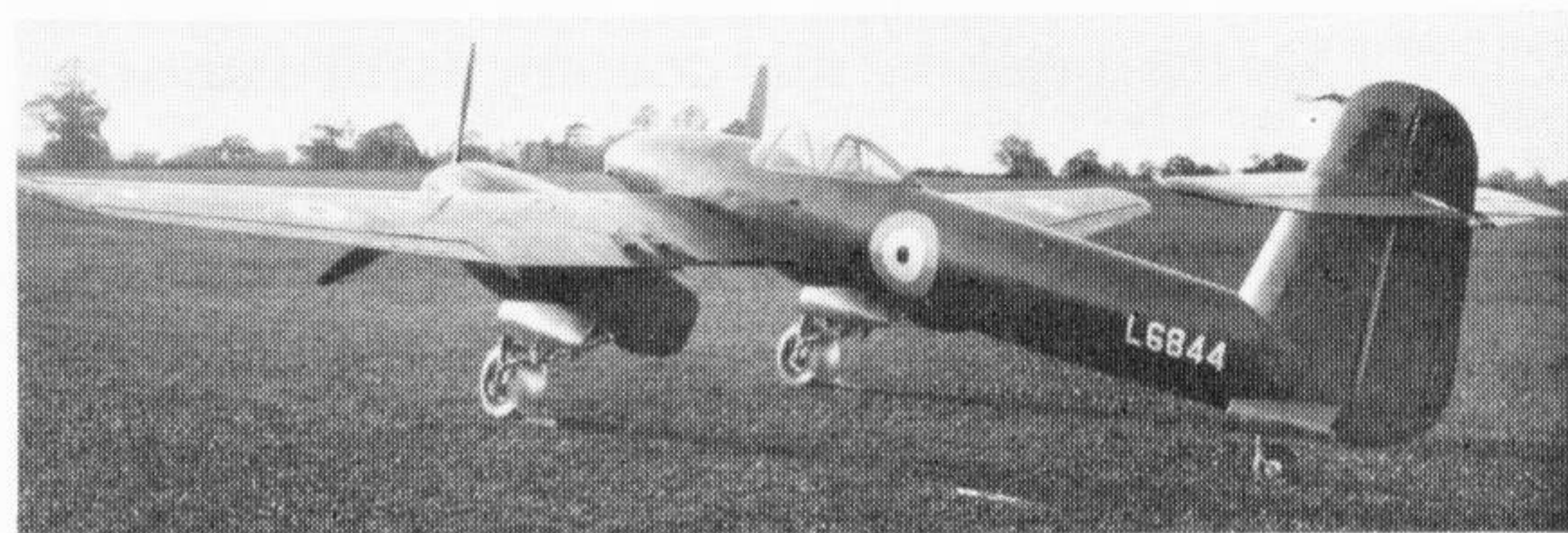
Three views of the first prototype, L6844, October 1938. Note girder bracing of front spar visible through intakes; also mudguards, and position of pitot head. Colour of L6844 was dark grey and NOT red, as is often stated.
