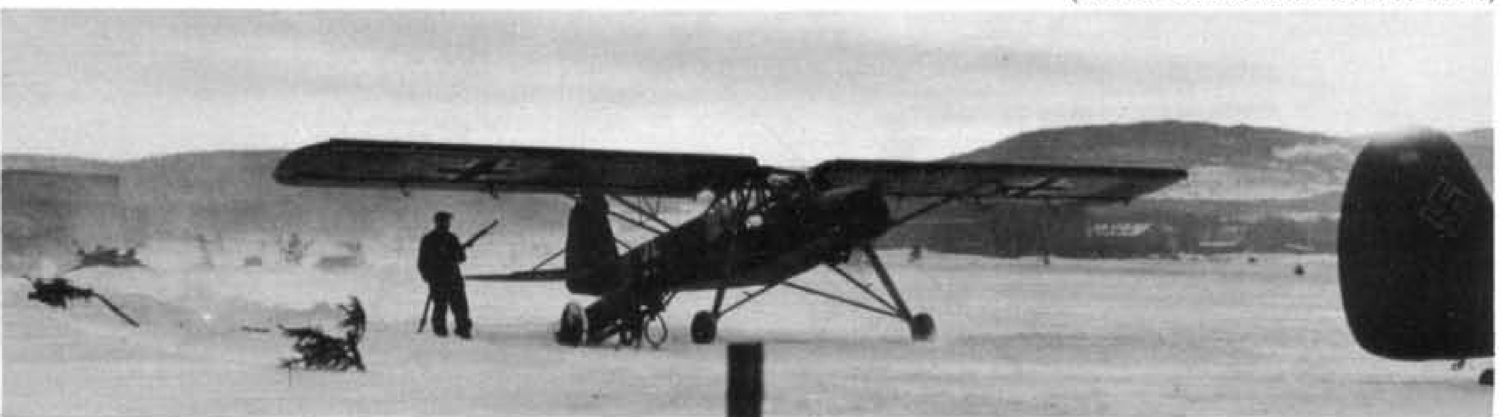
The versatile Storch could cope with quite severe snow before it was forced to exchange wheels for skis. Here a Fi 156 C is run up after being refuelled from an underground tank. This photograph was possibly taken at Kaufbeuren airfield in Bayern (Bavaria). (Photo: Bundesarchiv ref. 511-269-1)
