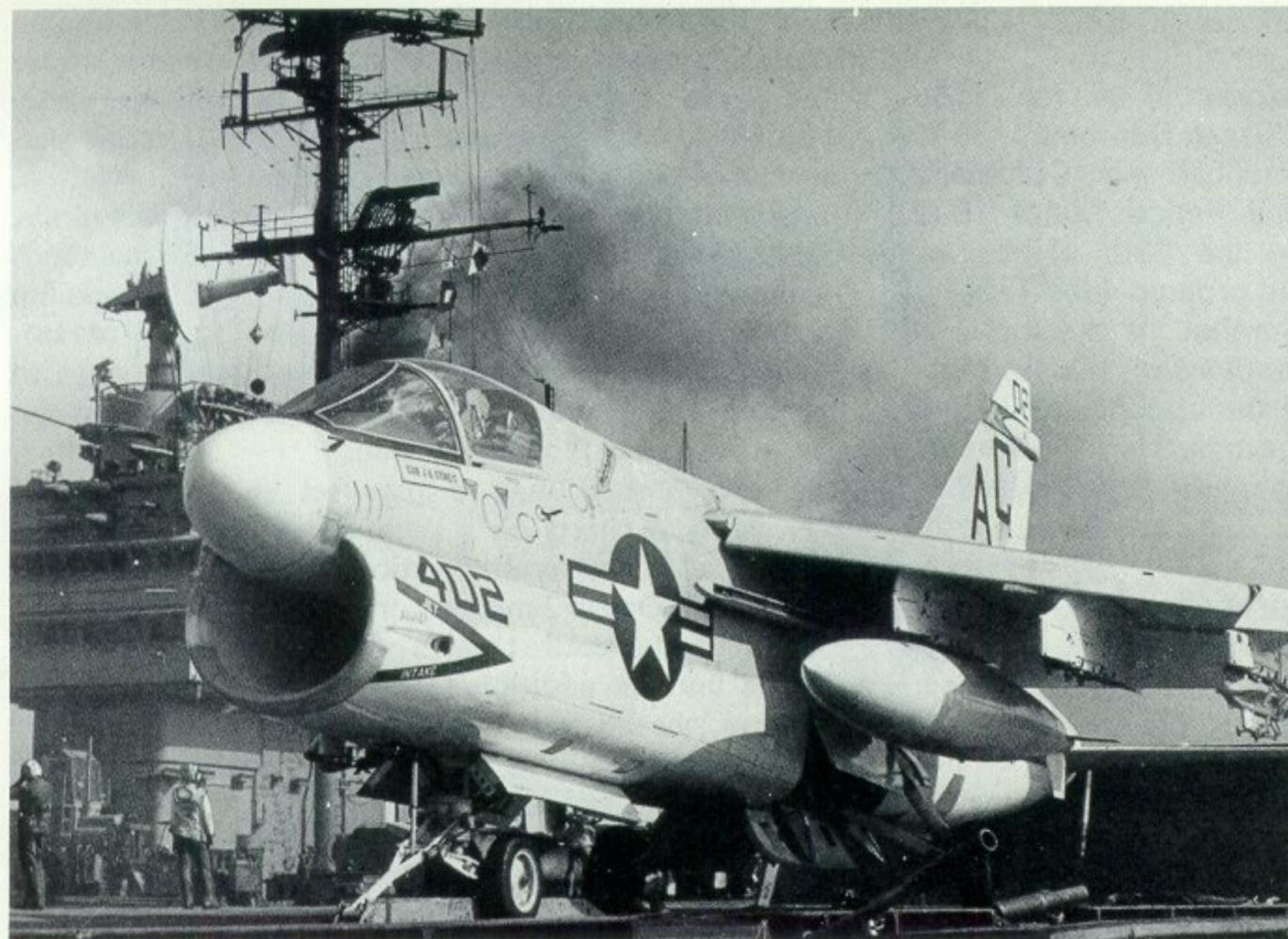
Aboard USS Saratoga in the Mediterranean 1969-70. An A-7B (BuNo. 154527) of the "Stingers", VA-113 of (AC) Carrier Air Wing Three. Commander J. B. Streit, USN, on the catapult. Bridle bar extending forward of nosewheel leg is neater arrangement than older catapult strop method. Wing leading-edge fully depressed. Drop tank holds 300-US gallons.
